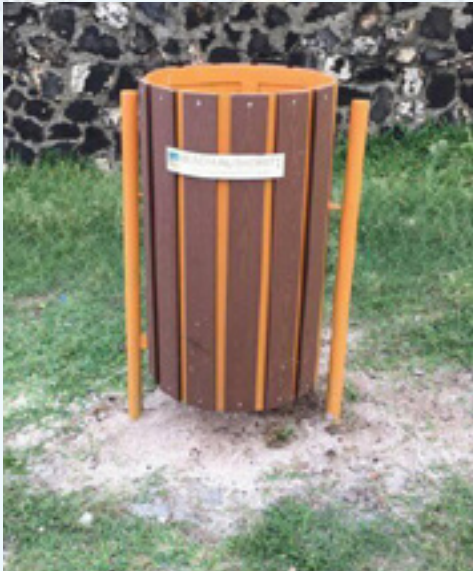
Litter bins made of galvanized iron sheets and cladded with wood composite plastic bars and fixed in reinforced concrete base at Roches Noires public beach
