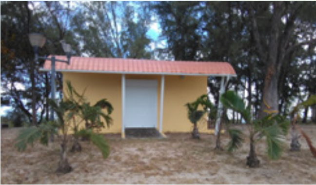
New toilet block at Pointe aux Piments public beach (near Cemetery)
