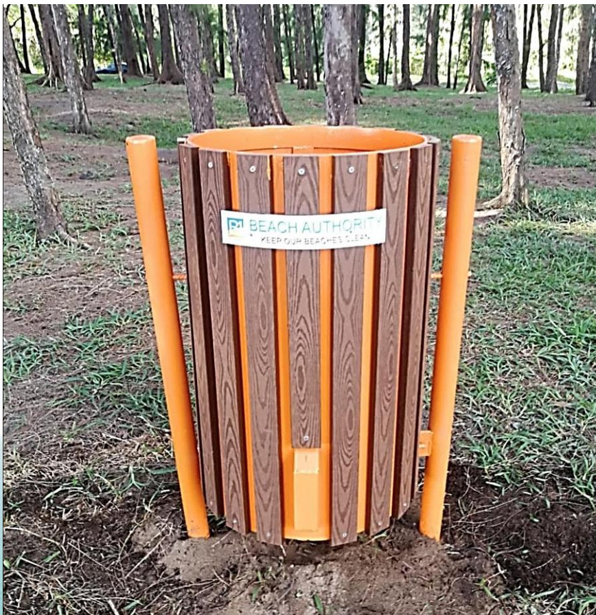
Litter bins made of galvanised iron sheets and cladded with wood composite plastic bars and fixed in reinforced concrete base at Le Bouchon public beach
