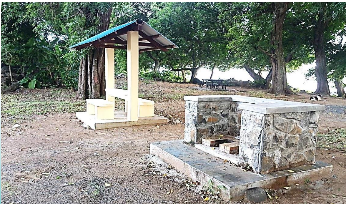
Provision of kiosk and fire place at Pointe des Lascars public beach
