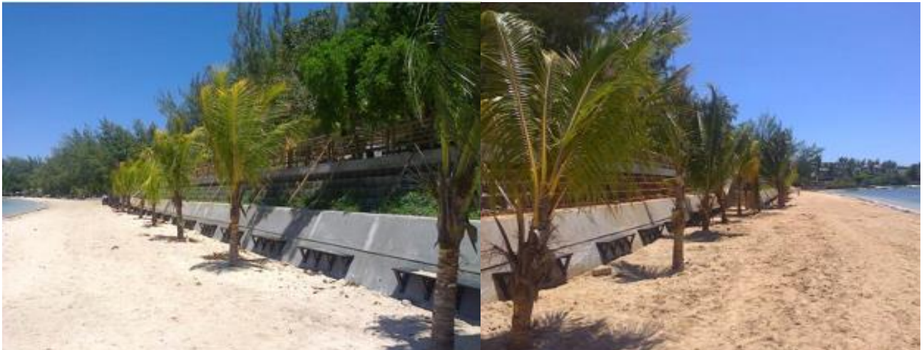
Fig 41: Terraced wall reconstructed, coconut trees planted and placement of plastic recycled benches at Bain Boeuf public beach
