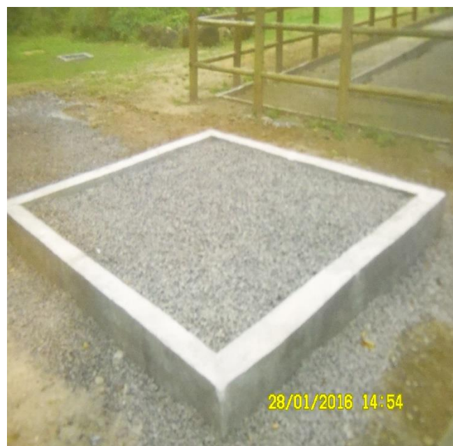
Fig 15: Construction of Absorption Pit
