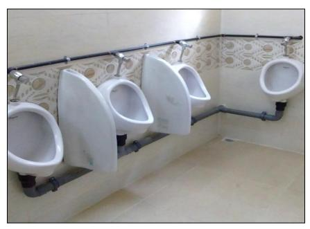
Supply and fixing of urinals with separators including bottle traps and flushing mechanism
