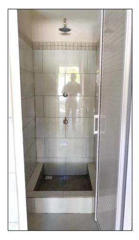
Supply and fixing of new shower head and tiling works
