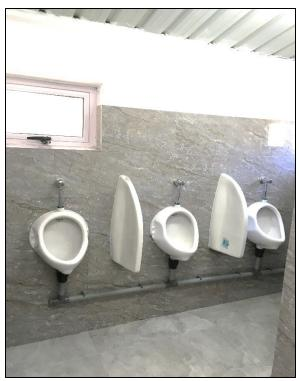
Supply and fixing of urinals with separators including bottle traps and flushing mechanism
