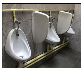
Supply and fixing of urinals with separators including bottle traps and flushing mechanism
