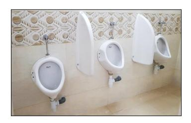
Supply and fixing of urinals with separators including bottle traps and flushing mechanism
