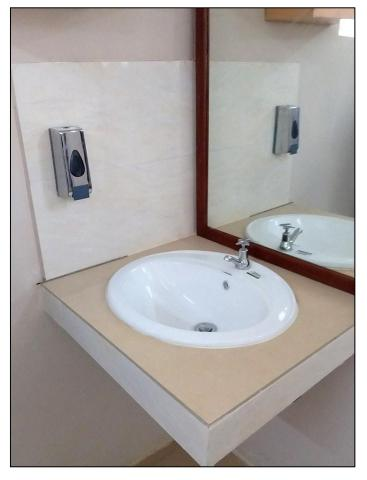
Fixing of wash hand basin mounted on a concrete platform and fixing of mirror
