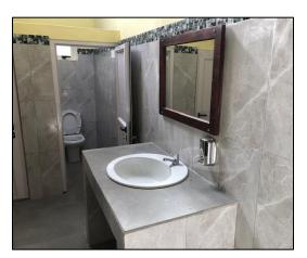
Fixing of wash hand basin mounted on a concrete platform and fixing of mirror
