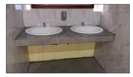
Supply and fixing of new wash basin mounted on a concrete platform
