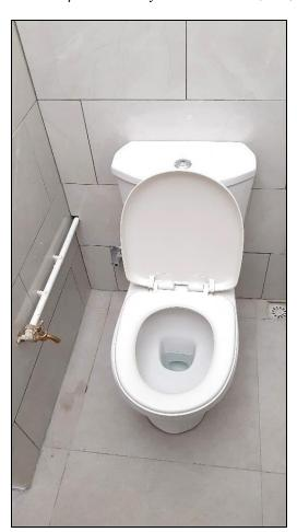
Supply and fixing of new Water Closet (WC) and tiling works
