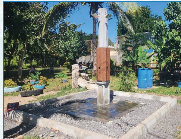
COMPLETED OPEN SHOWER AT TAMARIN PUBLIC BEACH
