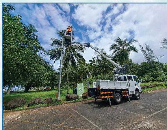
REPAIR OF EXISTING LIGHTING SYSTEMS USING LORRY WITH HYDRAULIC TELESCOPIC AERIAL PLATFORM AT ST FELIX PUBLIC BEACH
