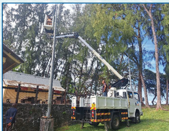
REPAIR OF EXISTING LIGHTING SYSTEMS USING LORRY WITH HYDRAULIC TELESCOPIC AERIAL PLATFORM AT ST FELIX PUBLIC BEACH
