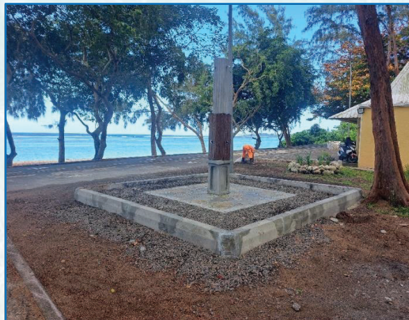
COMPLETED OPEN SHOWER AT ST FELIX PUBLIC BEACH
