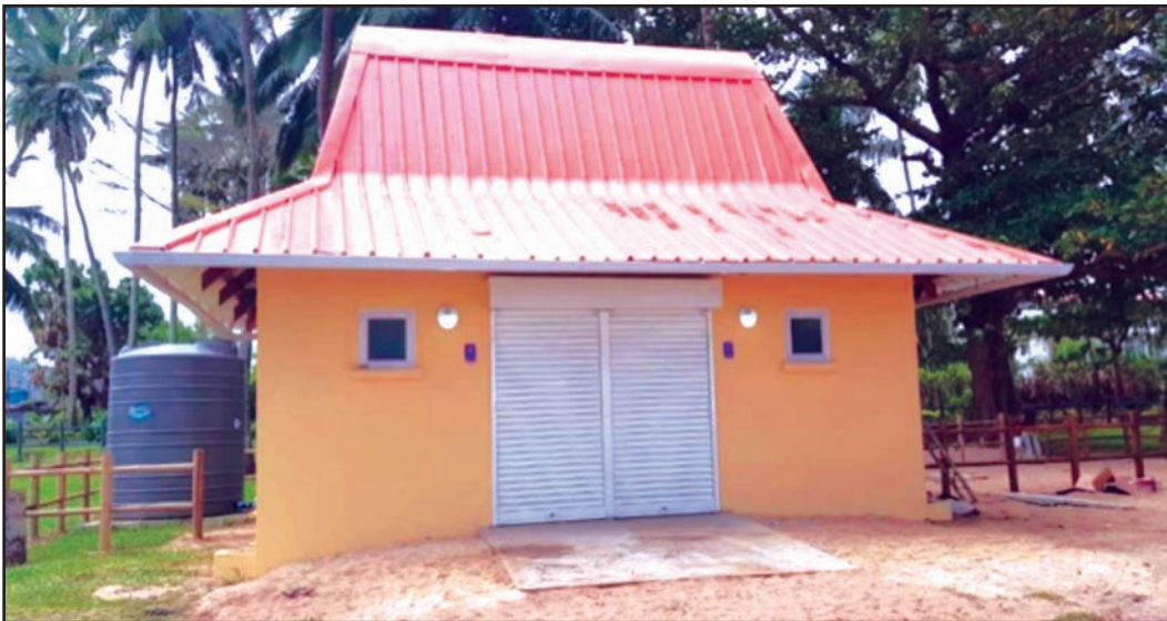
New toilet block at Riambel public beach
