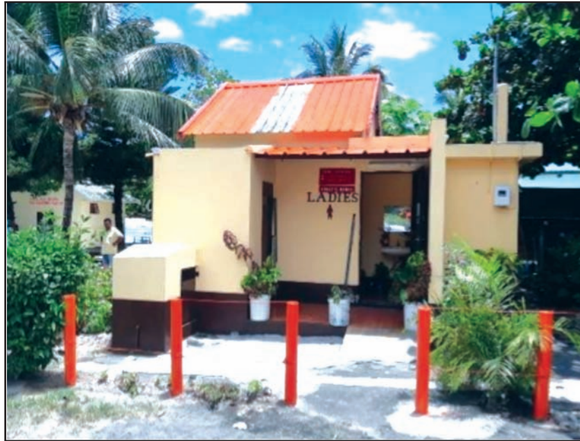
Upgraded of toilet block at Trou aux Biches (opp Ex- Aquarium) public beach
