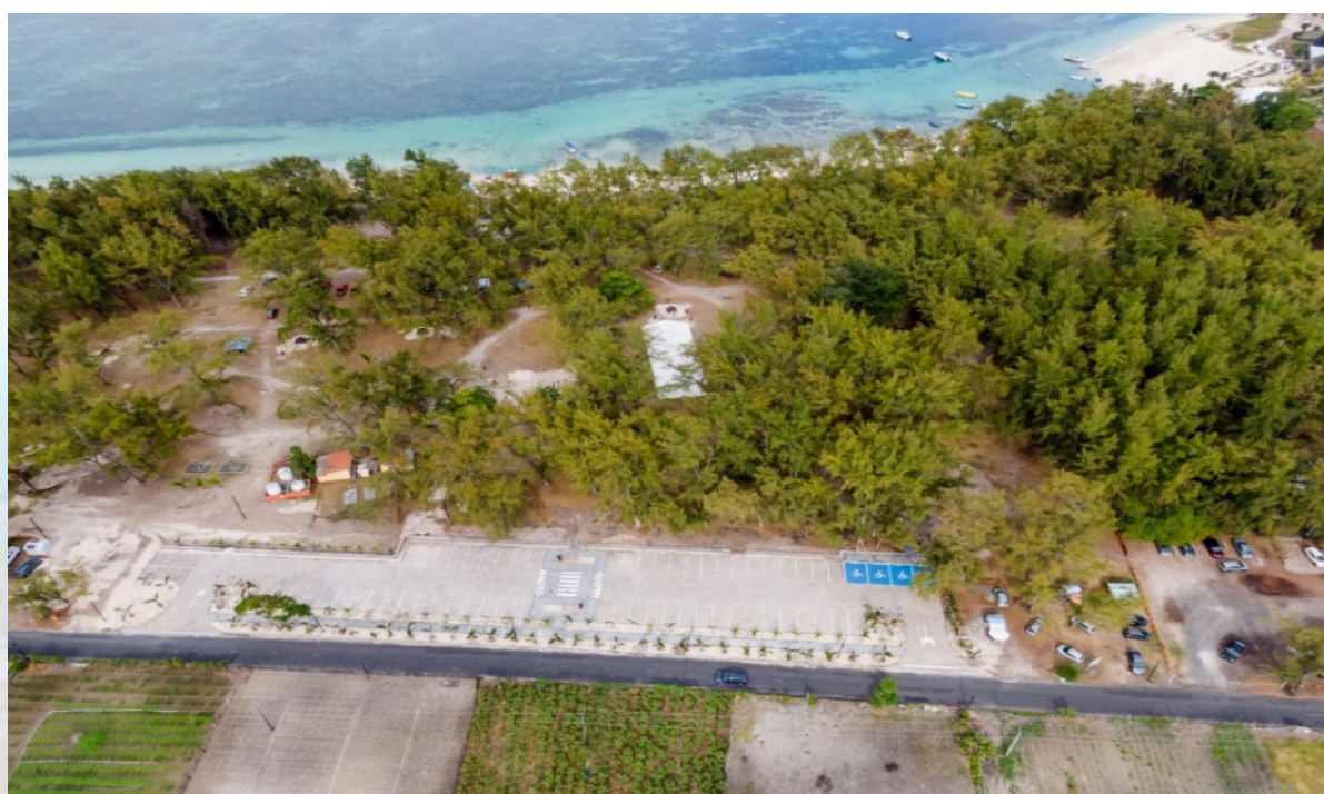
Aerials view of the refurbished parking at Belle Mare public beach
