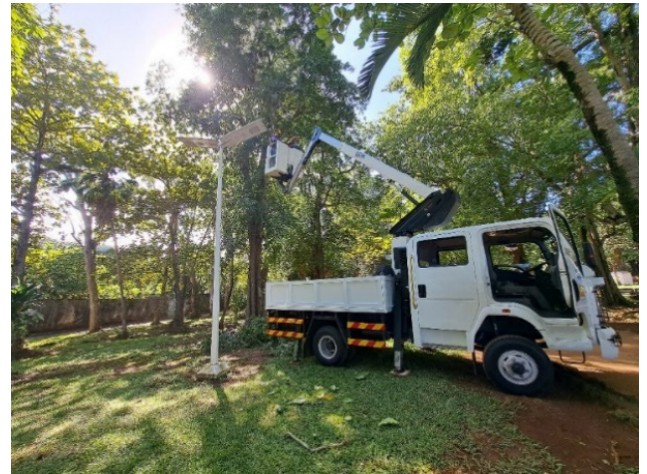
Repair of solar lighting systems and lopping of branches at Telfair & Gris Gris public beach using the double cab lorry with hydraulic aerial platform
