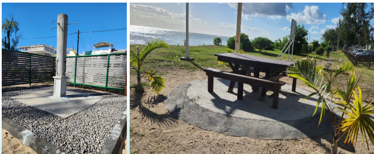
Construction of open shower and picnic tables
