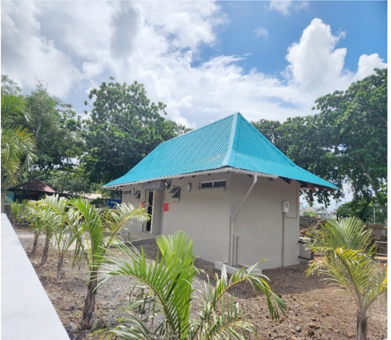
New Toilet Block at Blue Bay Public Beach
