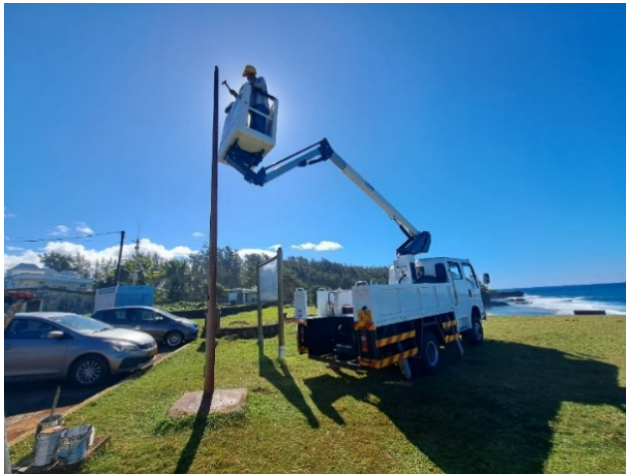
Repair of solar lighting systems and lopping of branches at Telfair & Gris Gris public beach using the double cab lorry with hydraulic aerial platform
