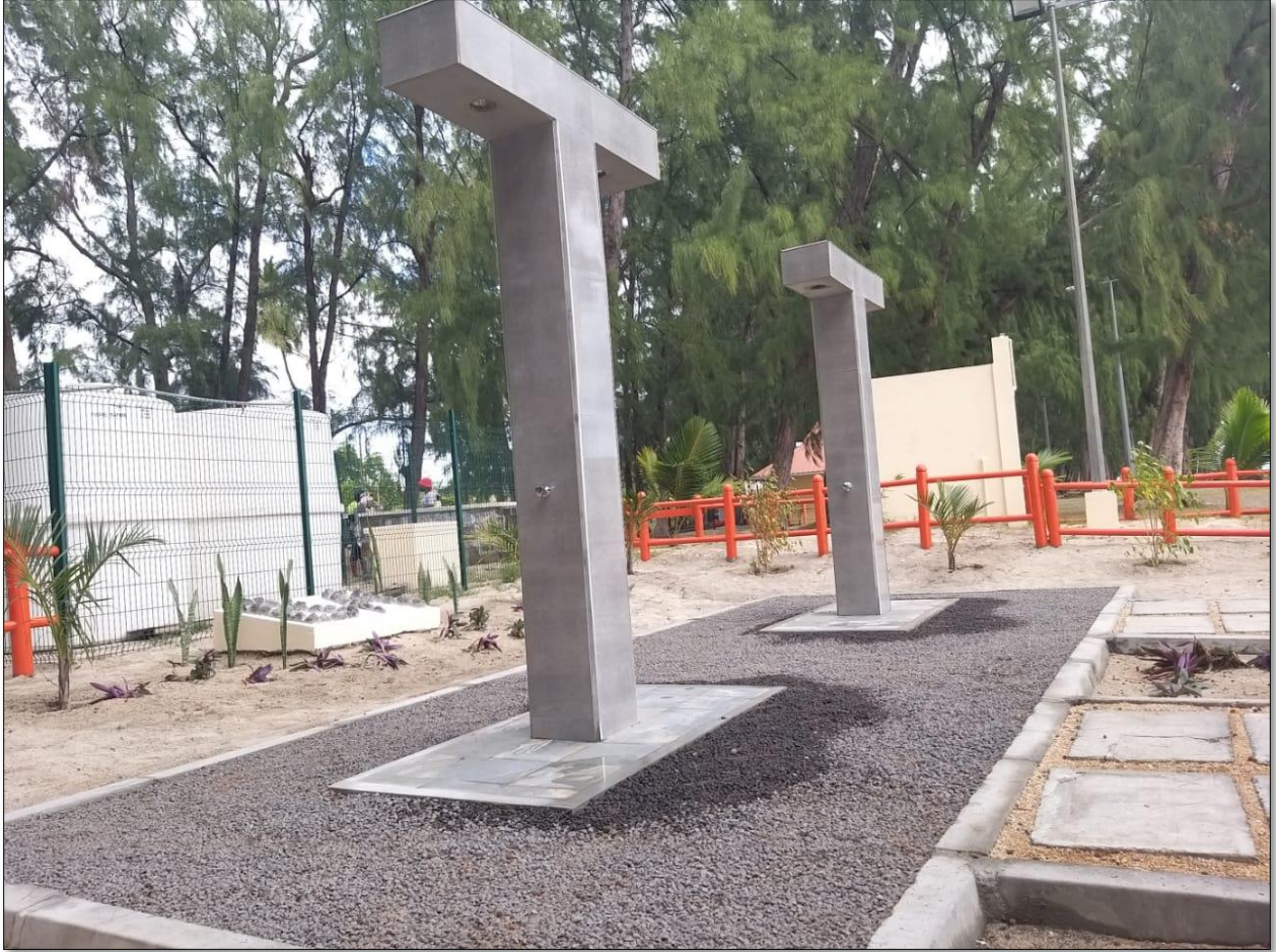
Construction of open shower – After
