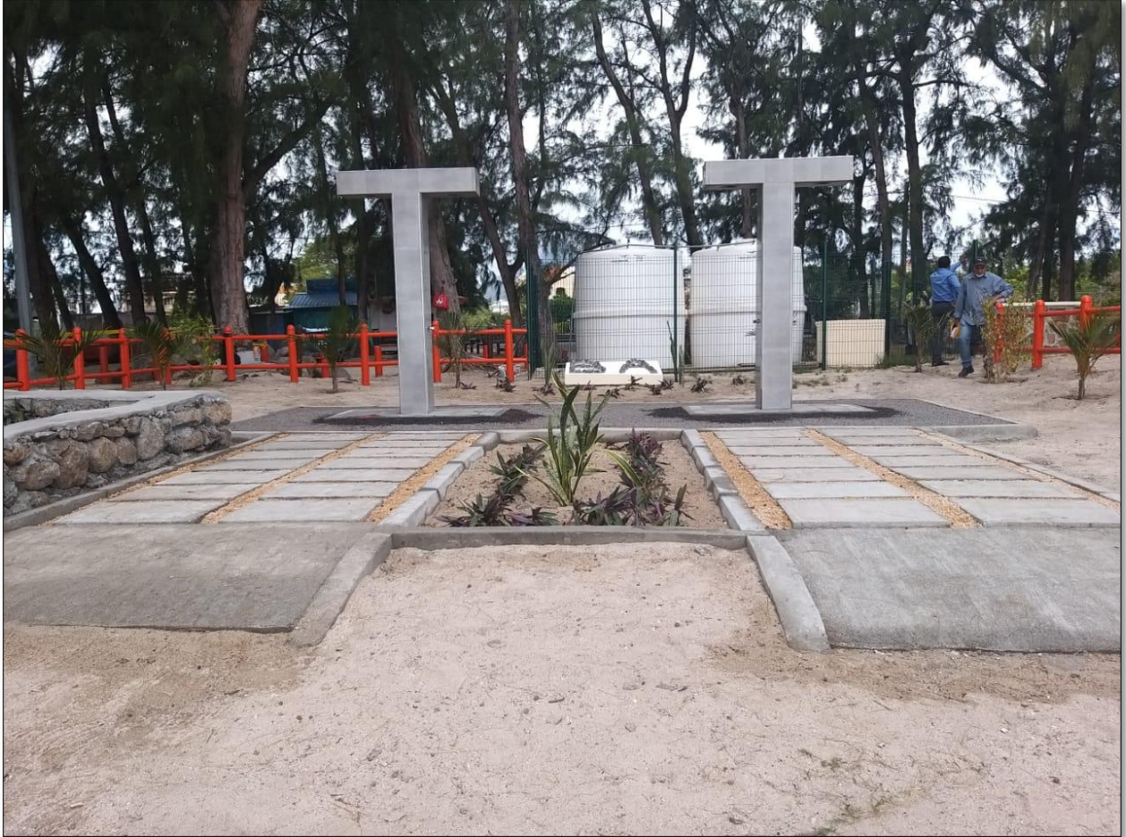
Enclosure of open shower and construction of access – After
