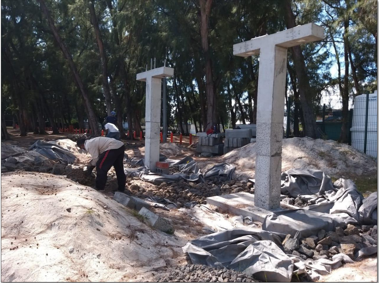
Construction of open shower – Before
