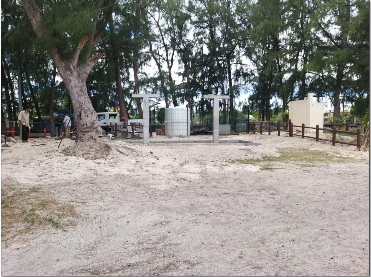
Enclosure of open shower and construction of access – Before
