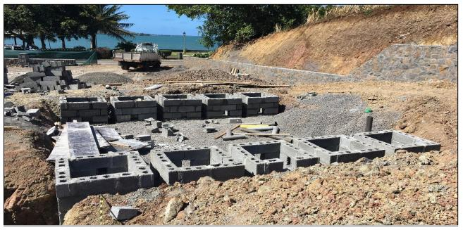
Excavation to receive components of leaching field is completed and construction of leaching field structure is ongoing
