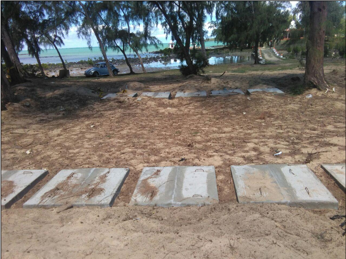
Construction of manhole covers
