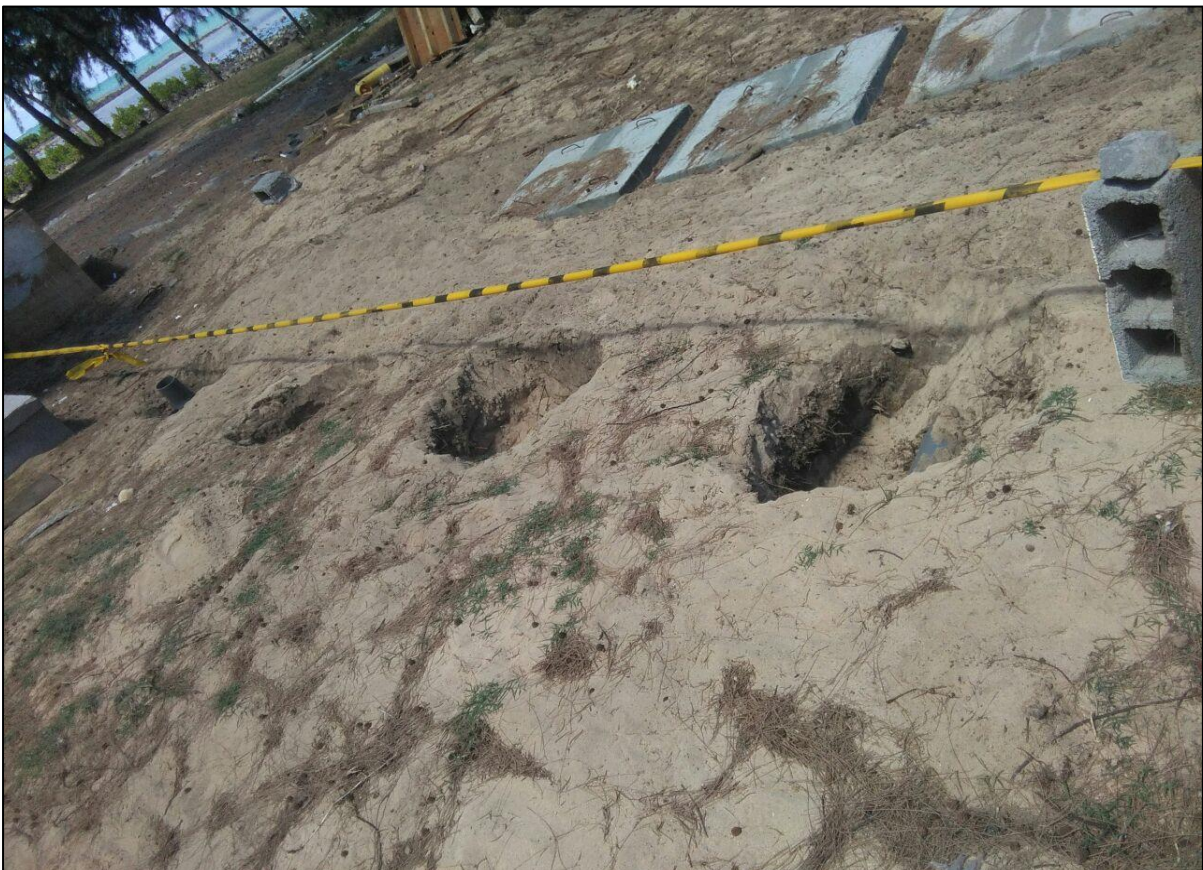
Excavation of wooden parapet enclosure for installation of pine poles
