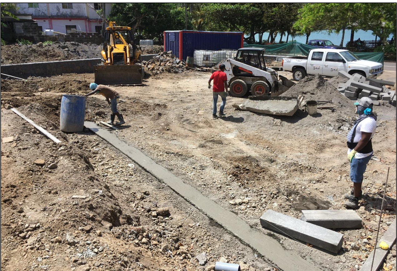
Haunching of kerbs surrounding the parking area is ongoing
