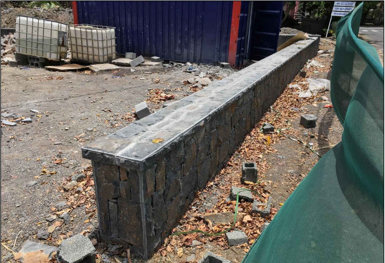
Construction of low stone masonry wall completed
