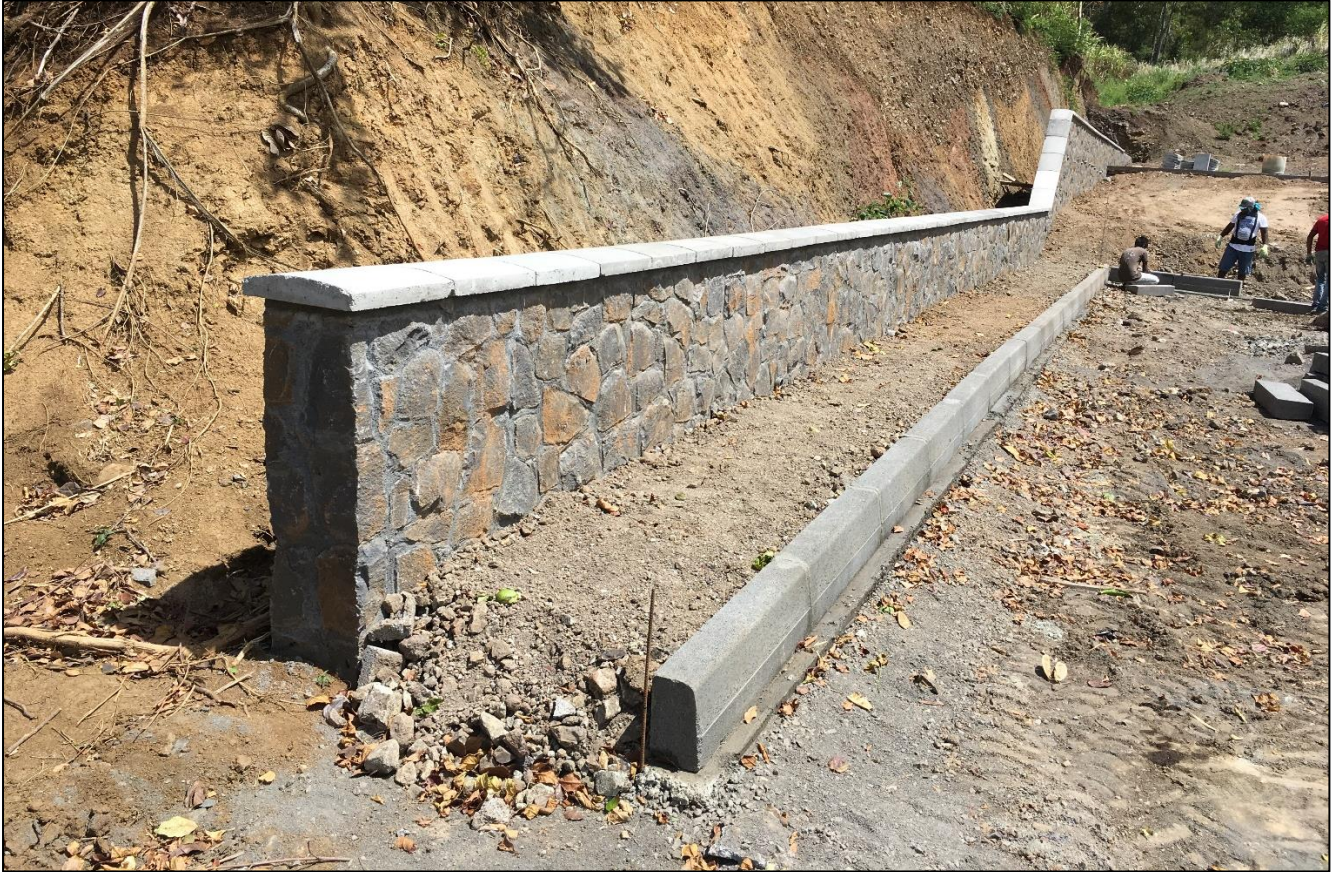
Coping work on retaining wall completed
