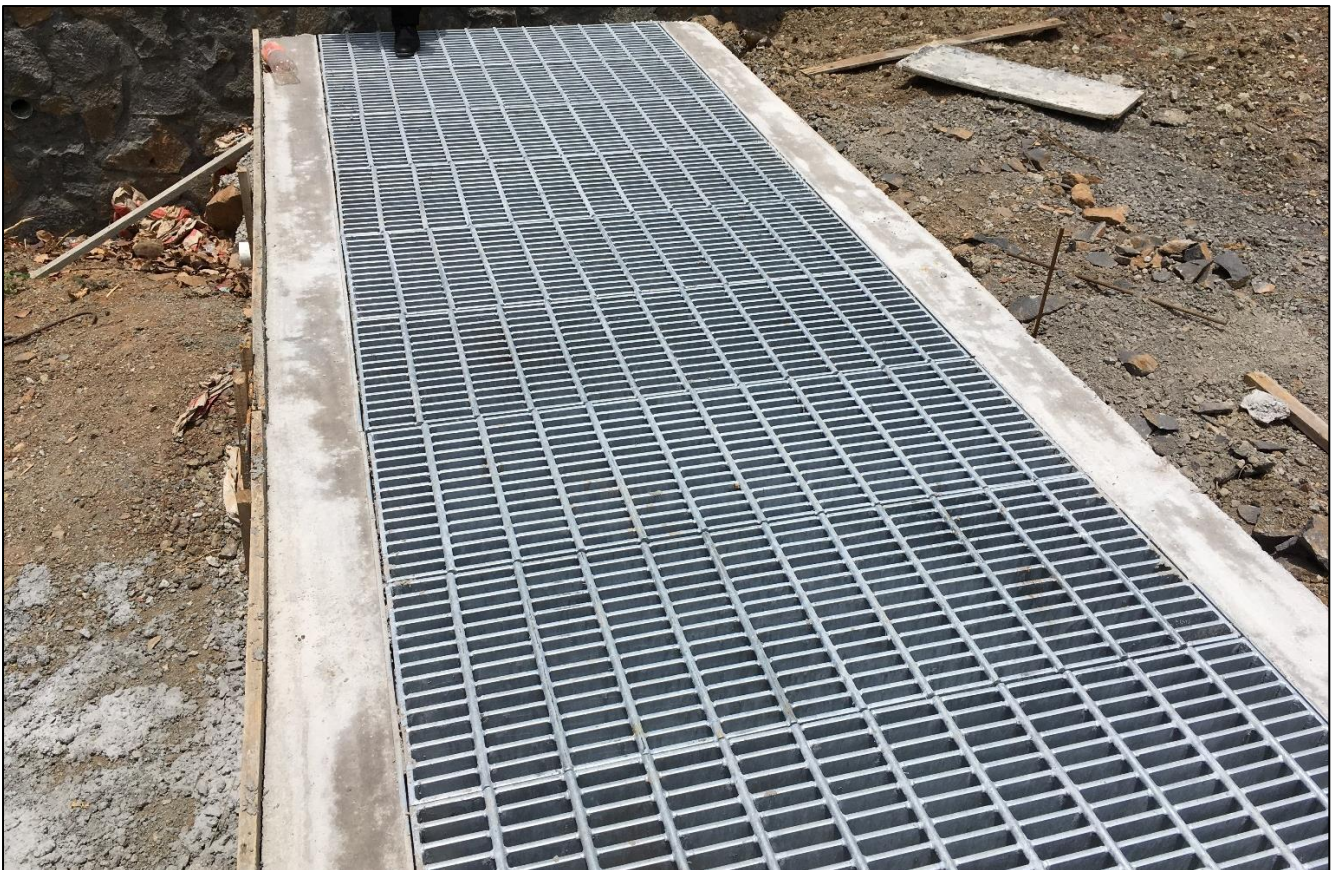
Metal grating on masonry drainage system completed
