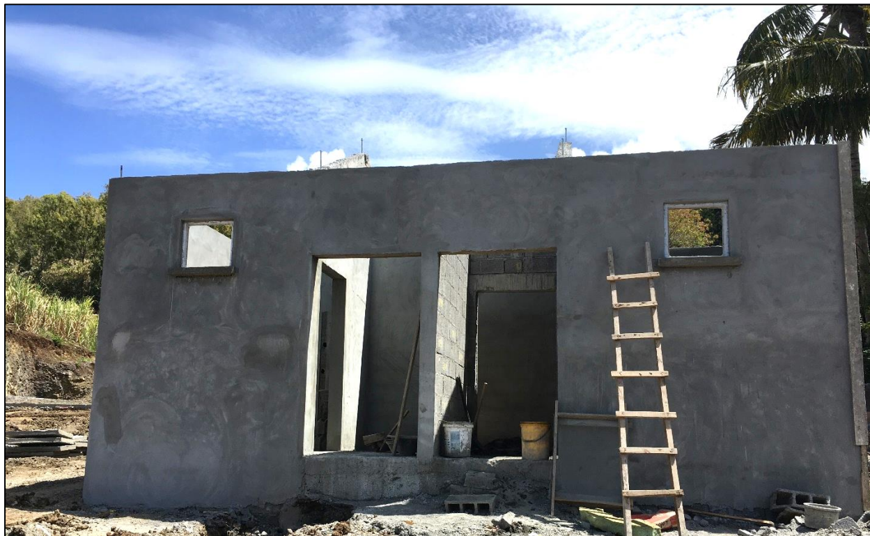
Erection of toilet blocks up to beam level completed and plastering work is ongoing
