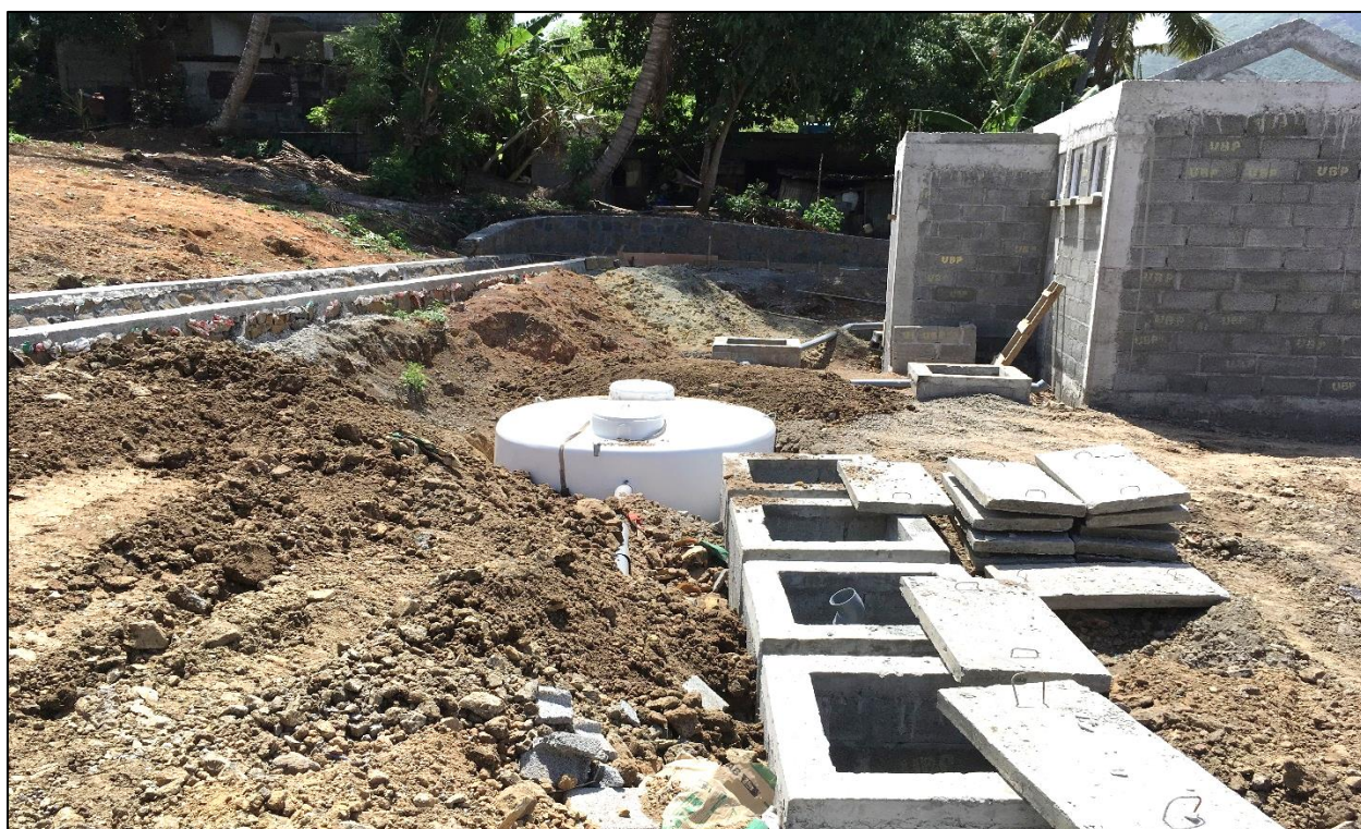
Installation and connections of new septic tank and construction of leaching fields
