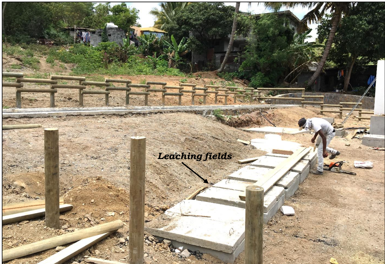
Enclosure of leaching fields with wooden parapet is ongoing
