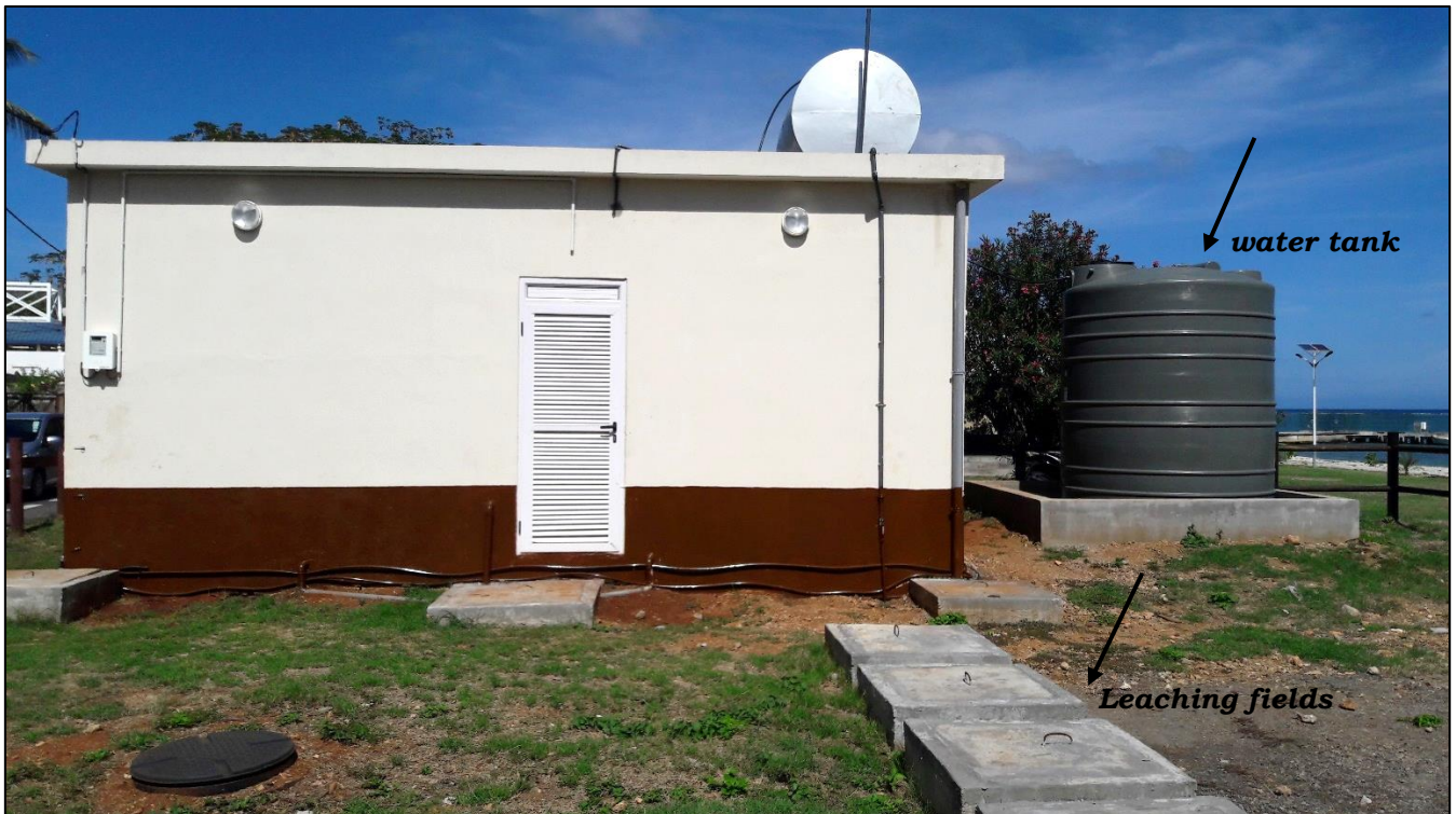
Provision of 9000 litres water tank and construction of new leaching fields
