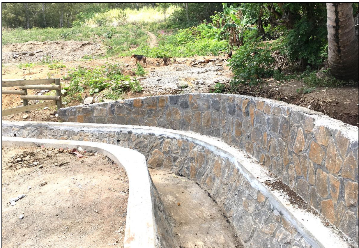
Construction of drainage system with blue basalt stone and concrete coping completed
