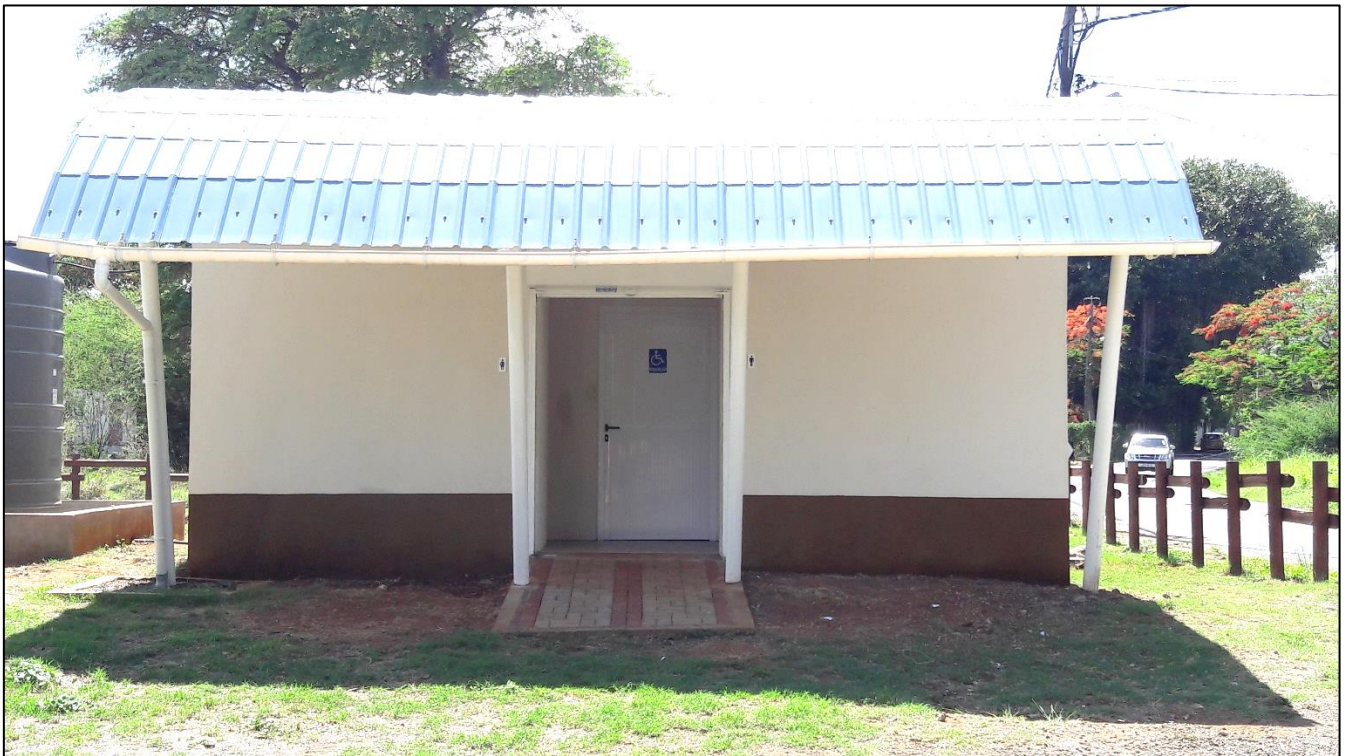
Painting of toilet blocks and fixation of Corrugated Iron Sheet (CIS) roof completed
