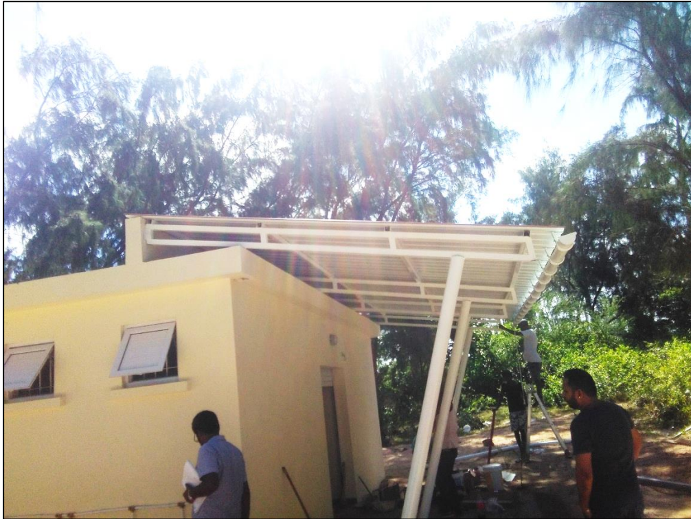
Fixation of Corrugated Iron Sheet (CIS) roof is ongoing
