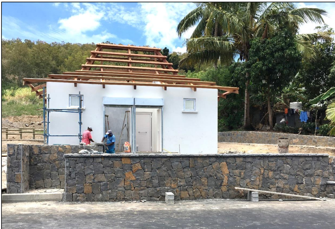
Construction of low masonry wall completed and construction of toilet blocks is ongoing
