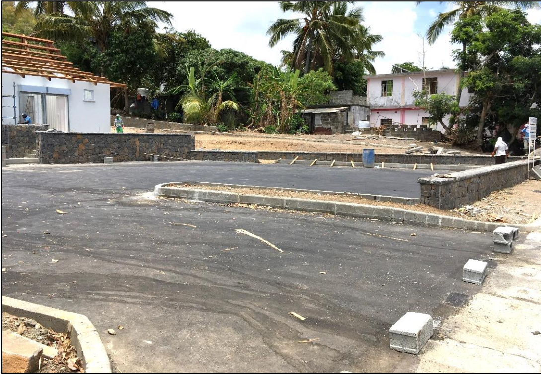
Asphalting of parking area completed and entrance has been lowered to facilitate vehicular access
