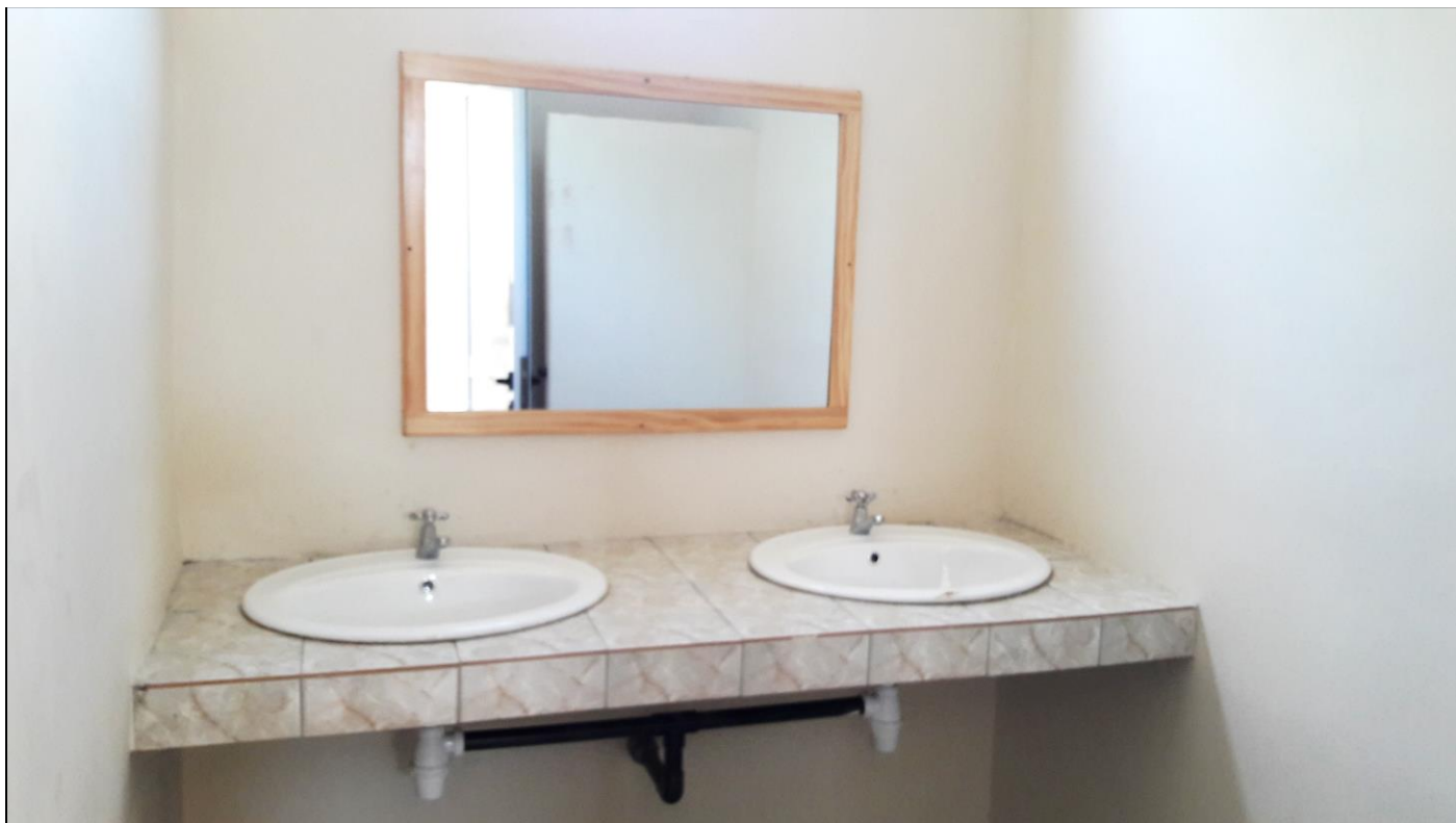
Fixing of wash basins mounted on a concrete platform and fixing of mirror
