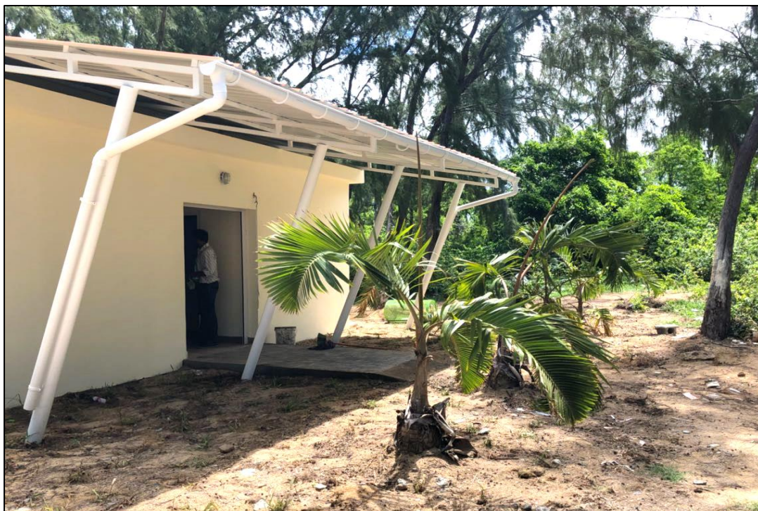
Painting of toilet blocks and fixation of Corrugated Iron Sheet (CIS) roof completed
