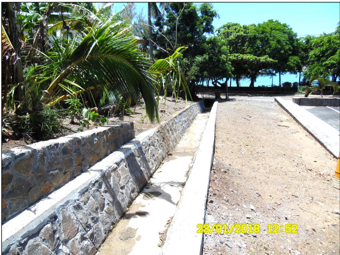
Construction of drainage system with blue basalt stone and concrete coping completed
