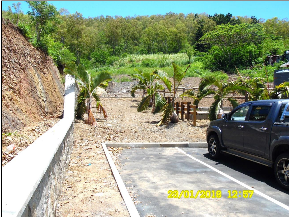
Coping work on retaining wall completed
