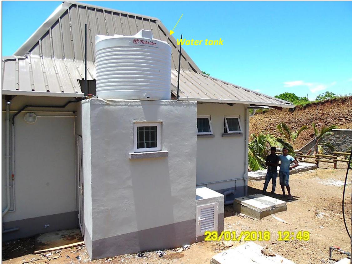
Provision of new water tank (2000 litres)
