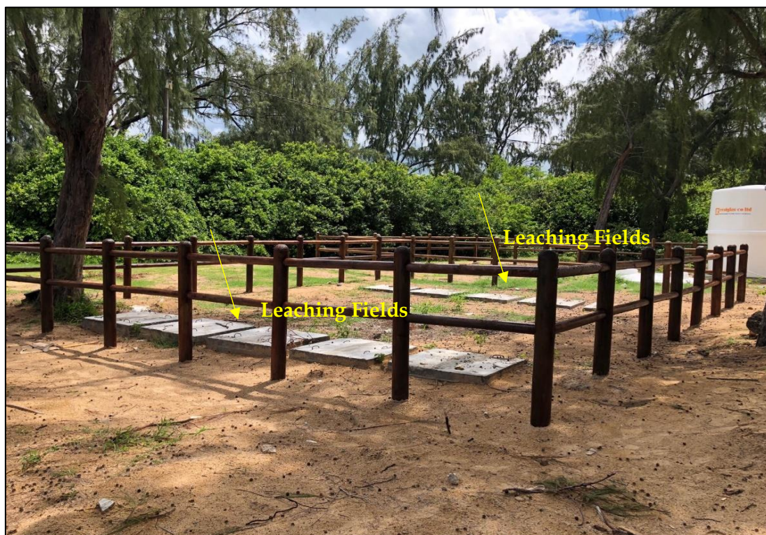
Enclosure of leaching fields with wooden pine poles
