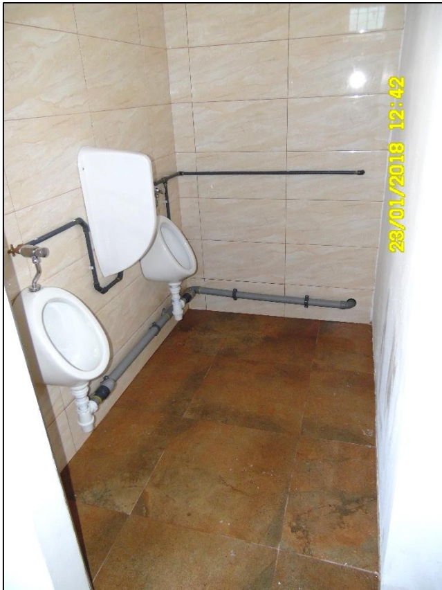
Supply and fixing of urinals
