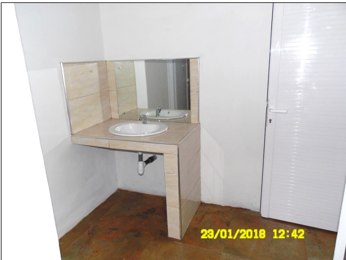
Fixing of mirror and wash basin mounted on a concrete platform
