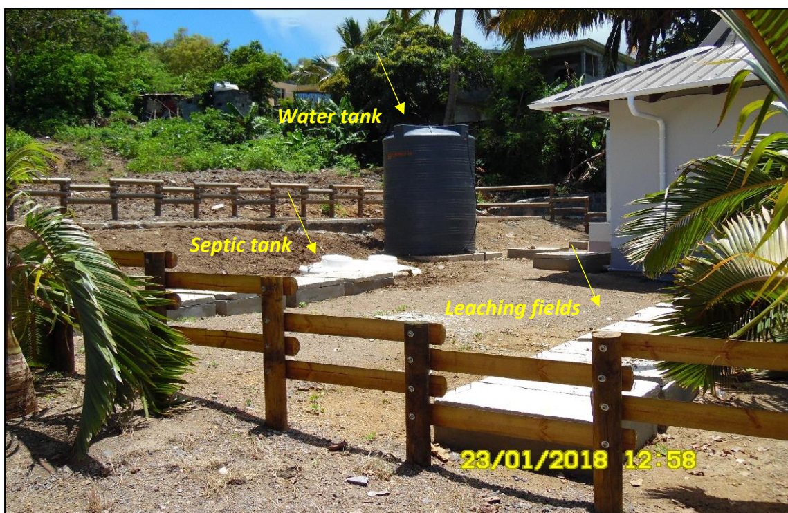
Enclosure of leaching fields, water tank and septic tank with wooden pine poles
