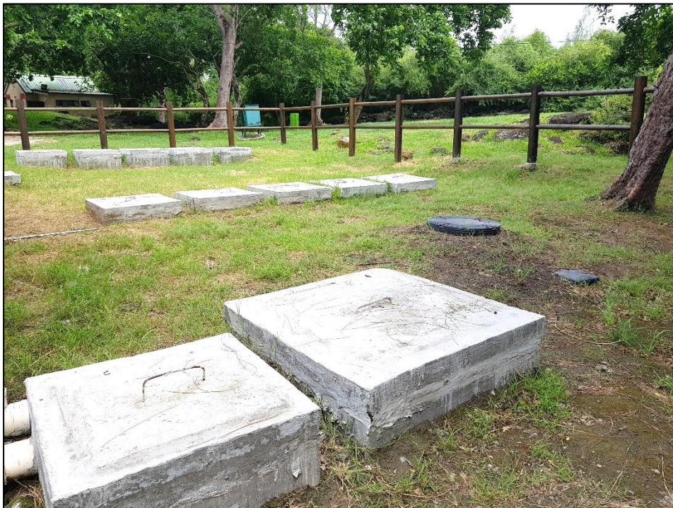
Enclosure of leaching fields with wooden pine poles
