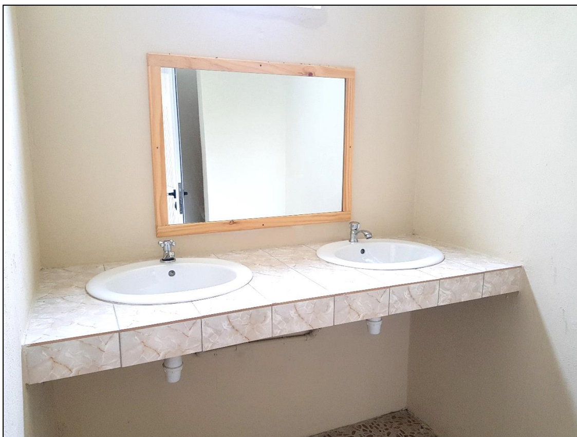
Fixing of wash basins mounted on a concrete platform and fixing of mirror
