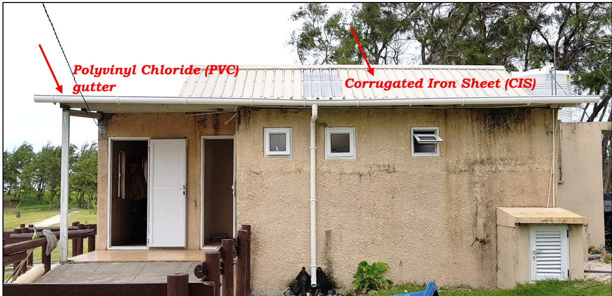
Replacement of Corrugated Iron Sheet (CIS) roof and Installation of Polyvinyl Chloride (PVC) gutter
