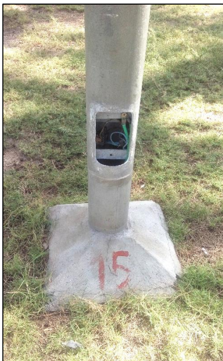
Tampering with the electrical system by beach users
