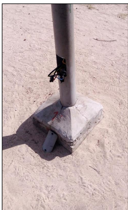
Tampering with the electrical system by beach users between 30.04.18 and 01.05.18
