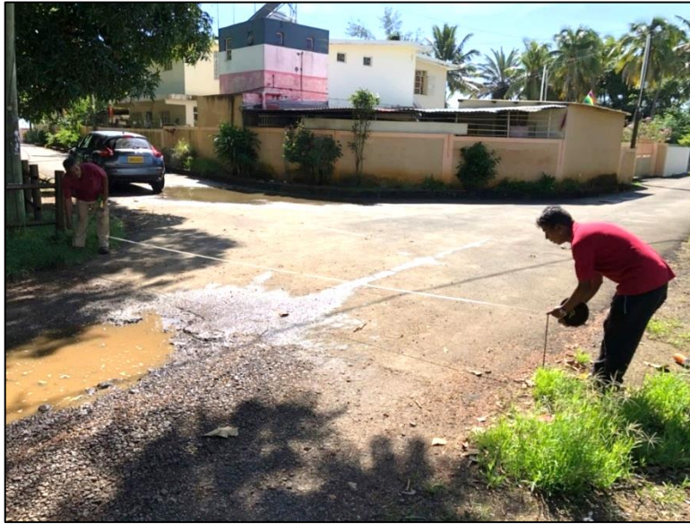
Setting out of parking boundary as per drawings
