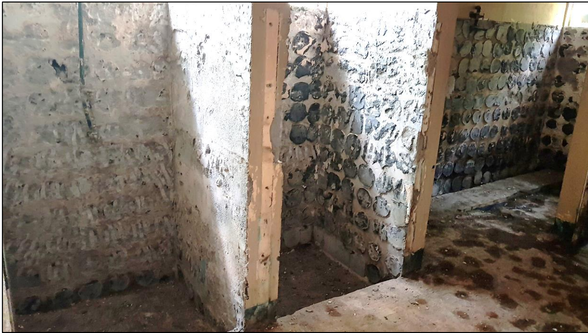
Removal of tiles completed
