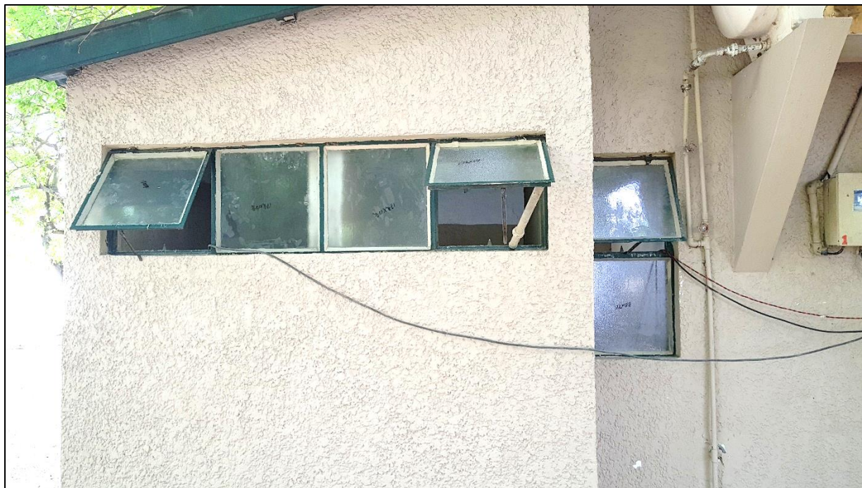
Reinstatement of existing window openings (ongoing)
