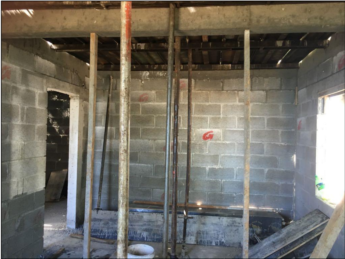
Shuttering works completed
