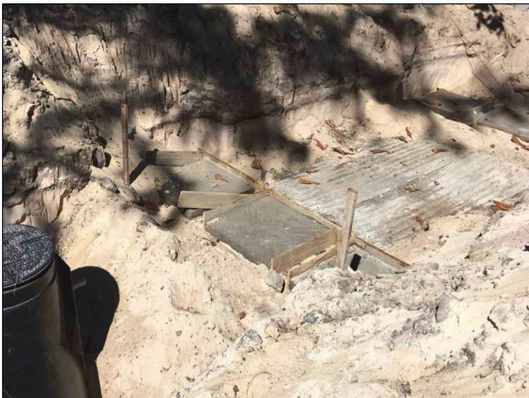
Construction of leaching field is ongoing
