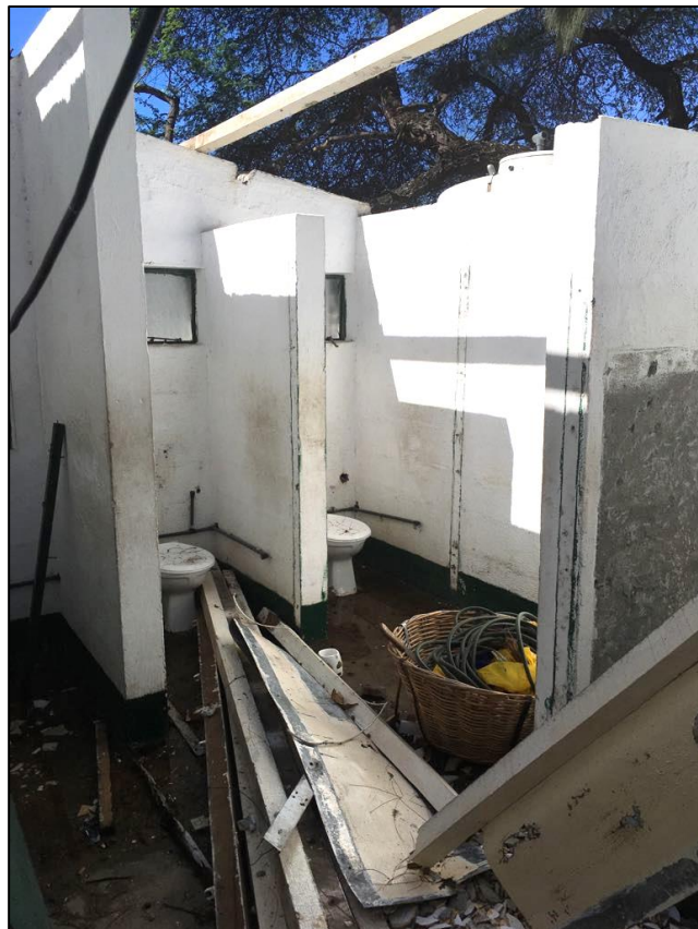
Removal of roof sheeting, wooden purlins and rafters (to be replaced by new ones shortly)
