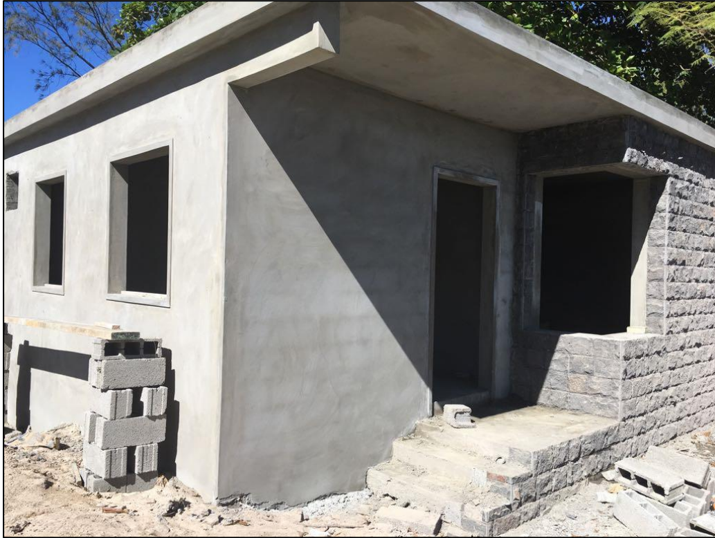
Interior and exterior plastering works and cladding wall with blue basalt stones completed
