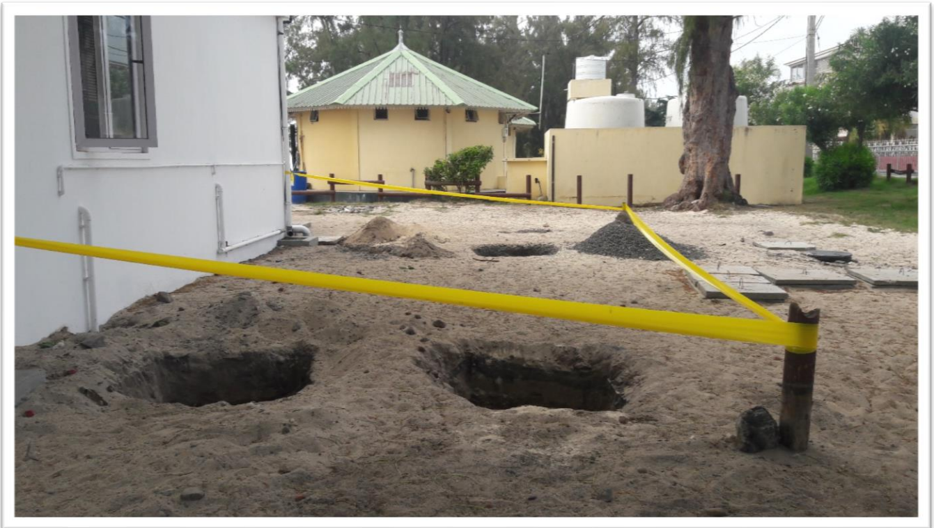
Excavation for casting of concrete base
