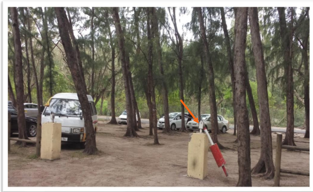
Lever- arm damaged by vandals
