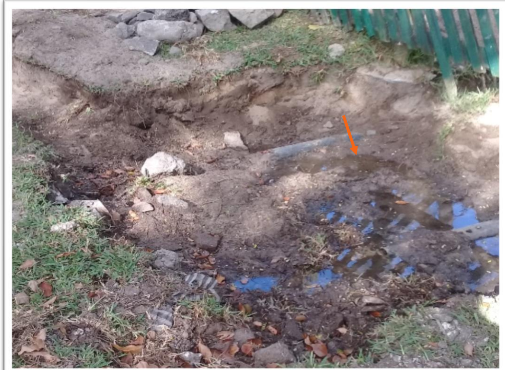
Clogged absorption pit at La Cuvette public beach
