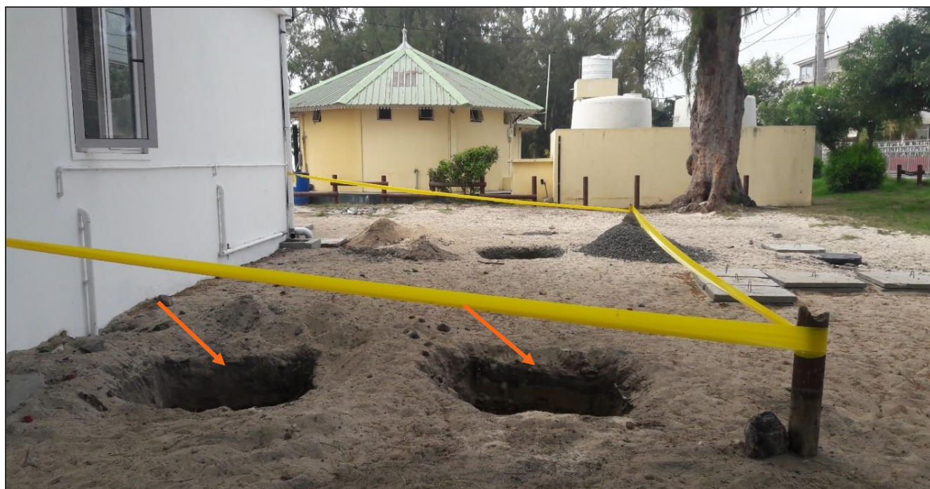
Excavation works for casting of concrete base for placing of container
