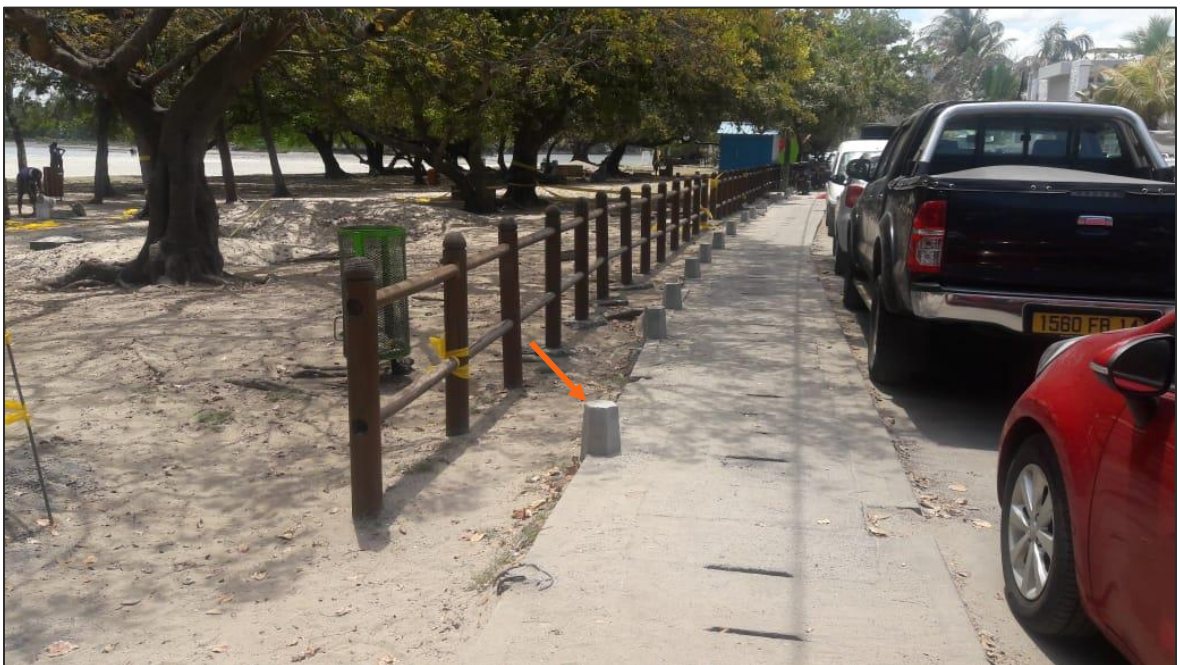
Reinstatement of existing concrete bollards in progress
