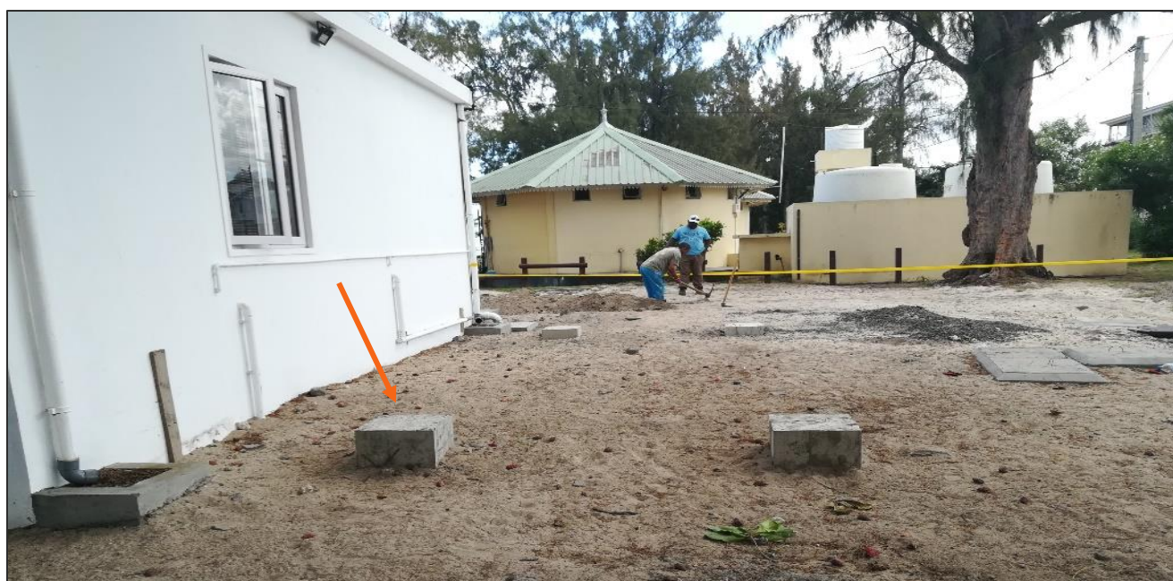
Concrete base for container already casted
