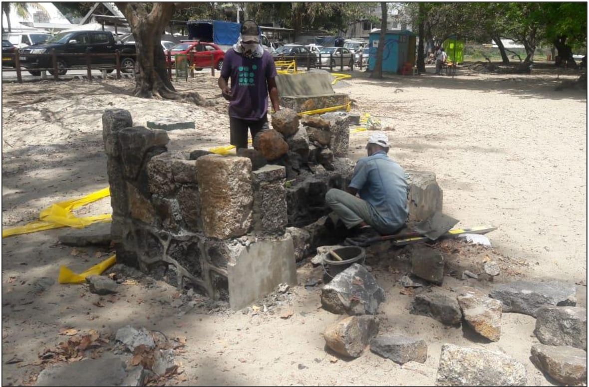
Upgrading works of existing stone masonry fireplace in progress
