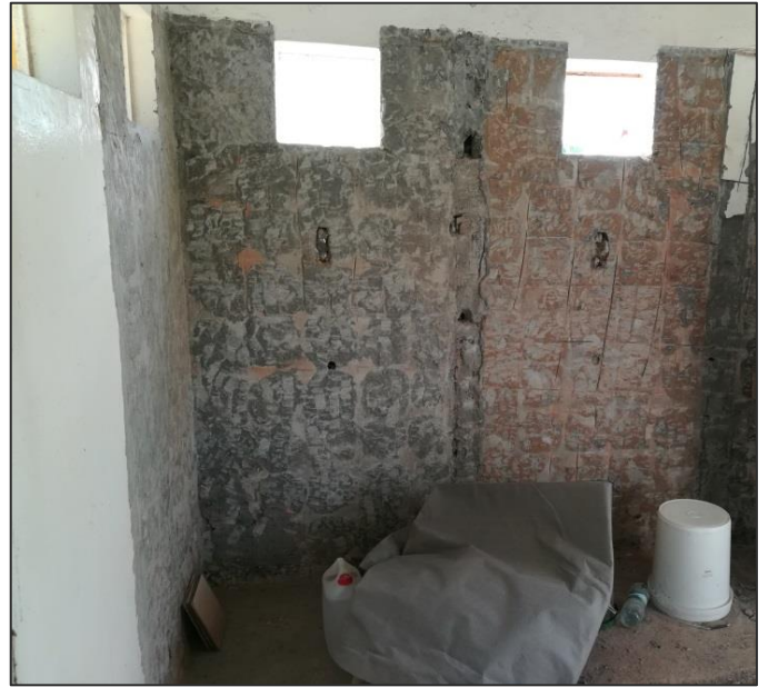
Removal of existing tiles of Commercial Building at Blue Bay public beach
