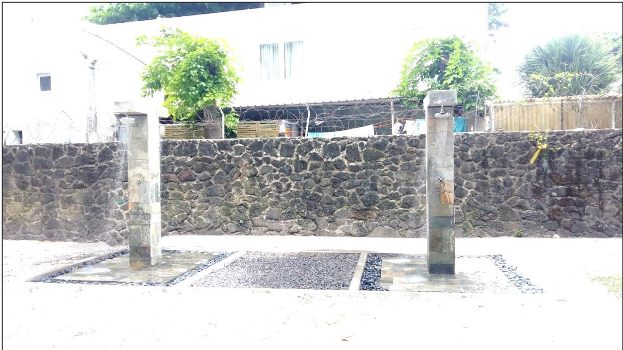
Newly constructed open showers at Pereybère public beach (completed in December 2018)
