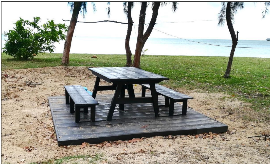
Supply and installation of four (4) picnic tables at P.G L'Embrazure public beach
