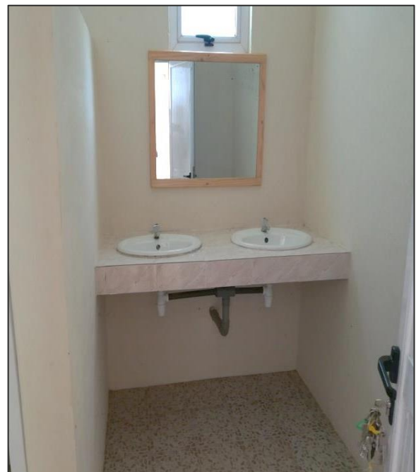
Fixing of wash hand bassins mounted on a concrete platform and fixing of mirror
