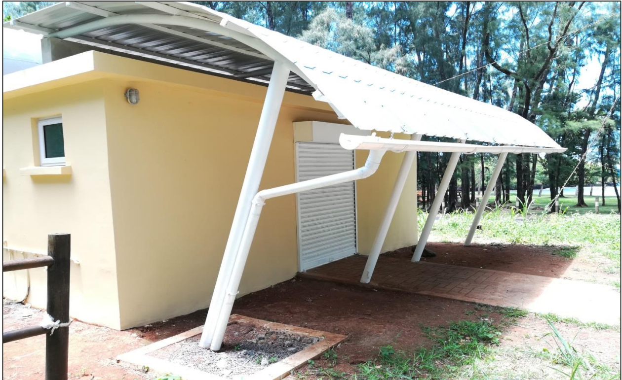
Painting of toilet blocks and fixation of Corrugated Iron Sheet (CIS) roof completed
