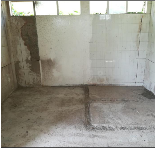
Removal of existing tiles of Commercial Building at Blue Bay public beach
