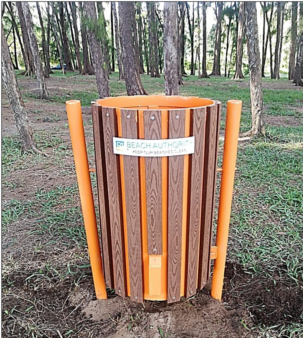
Litter bins made of galvanised iron sheets & cladded with wood composite plastic bars and fixed in reinforced concrete base at Pomponette public beach
