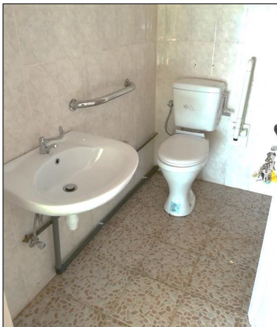
Provision of toilet for disabled persons
