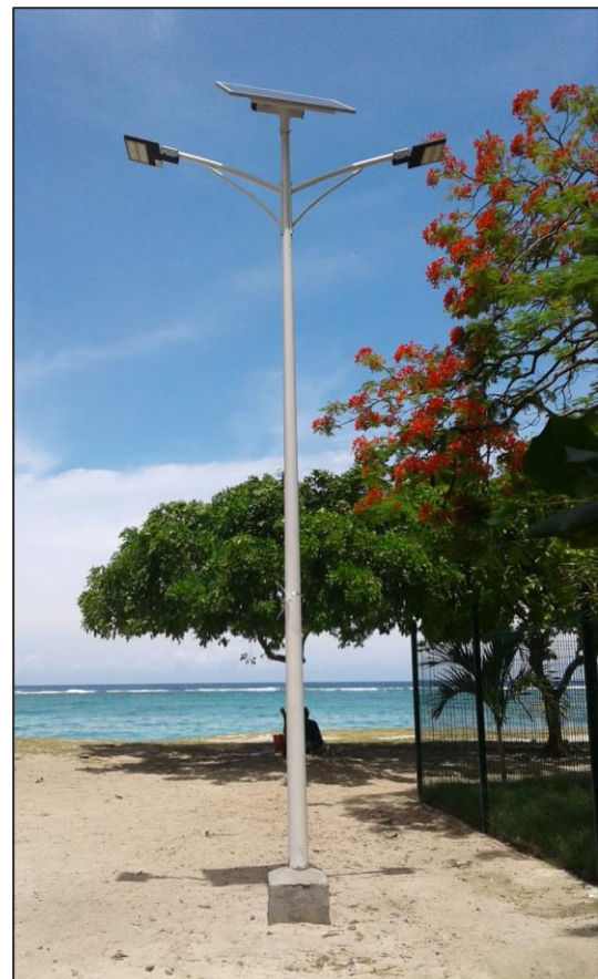
New lighting facilities through PV Solar Panels at Flic en Flac public beach
