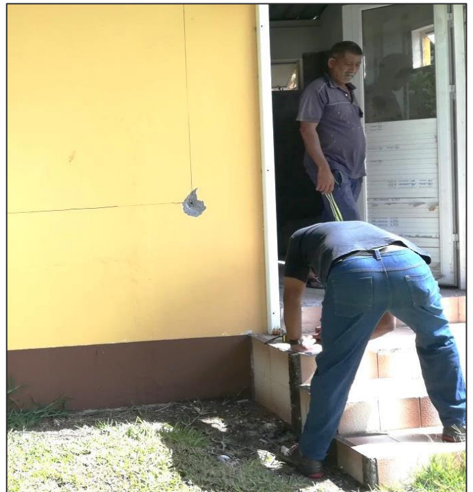
Provision of aluminium door openings for Commercial Building at Blue Bay public beach (Ongoing)
