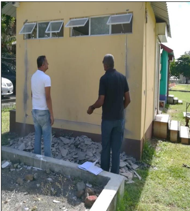
Construction of waste water disposal system for Commercial Building at Blue Bay public beach (Ongoing)
