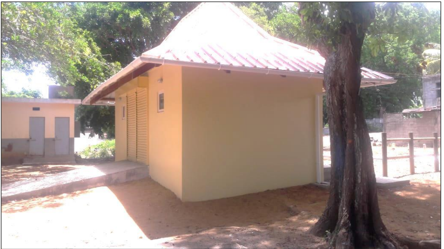
Newly constructed Toilet Blocks at Pointe des Lascars public beach
