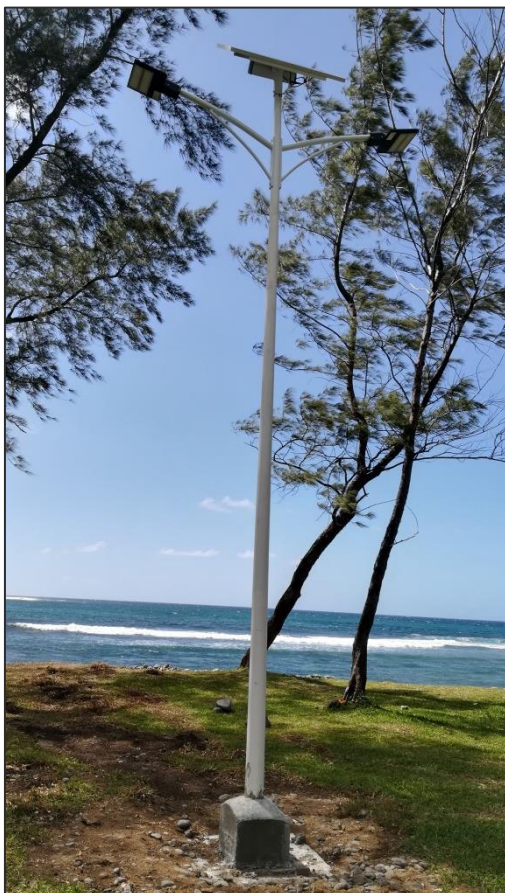
New lighting facilities through PV Solar Panels at Rivière des Galets public beach
