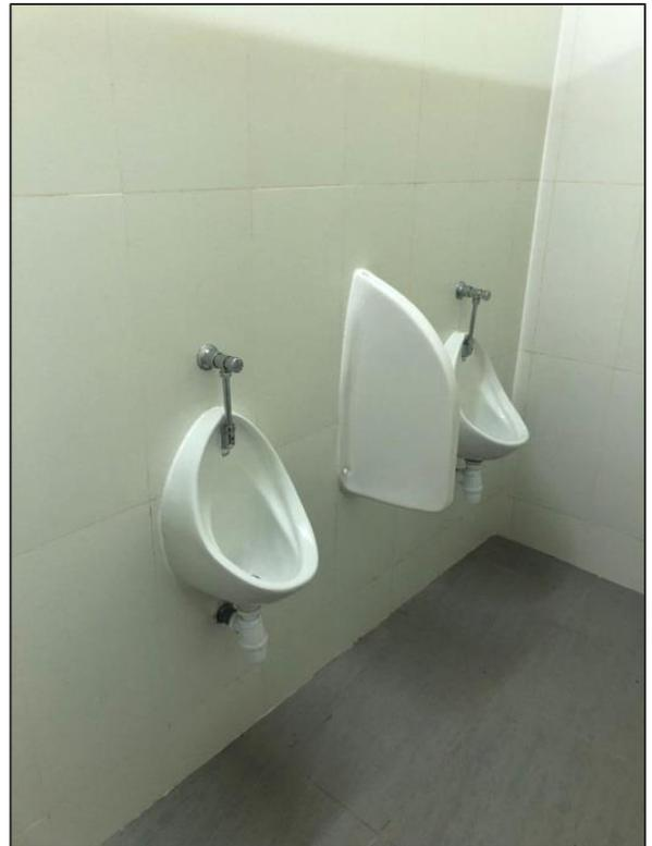
*Supply & fixing of urinals with separators including bottle traps and flushing mechanism*
