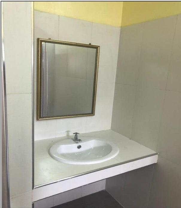
*Fixing of wash hand basin mounted on a concrete platform and fixing of mirror*
