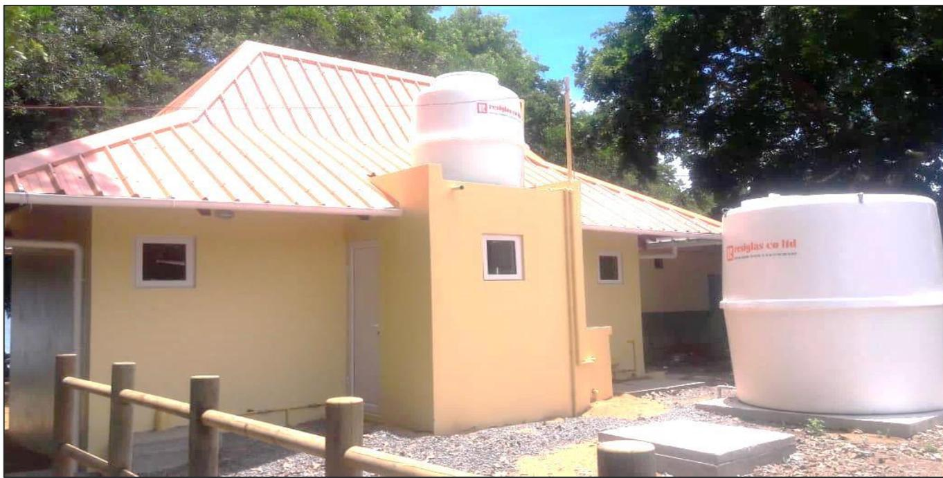
*Newly constructed Toilet Blocks at Pointe des Lasars public beach equipped with 9000 L water tank, septic tank and leaching field*
