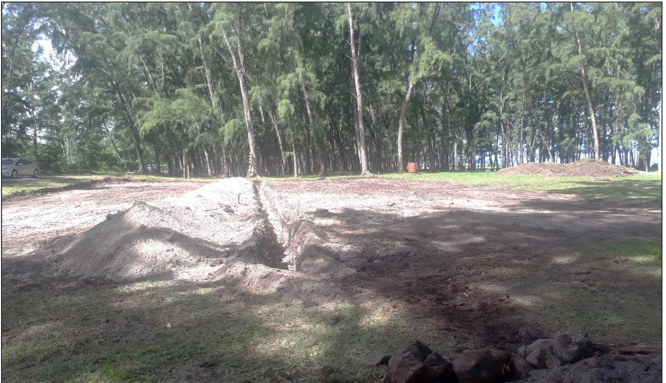
*Removal of top soil and excavation of trench for french drain completed at Pomponette public beach*
