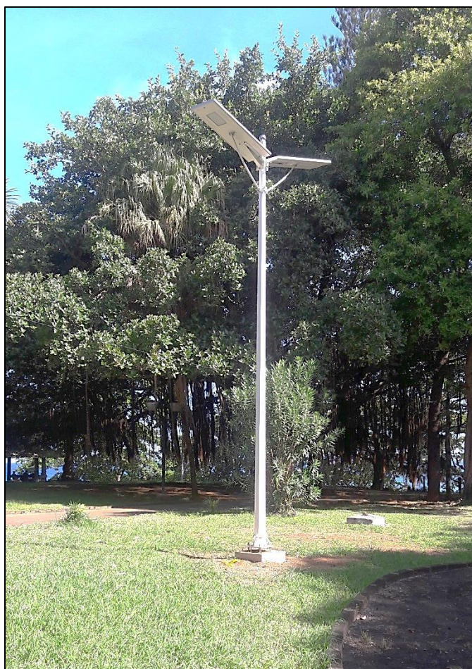
Solar lighting system at Telfair public beach
