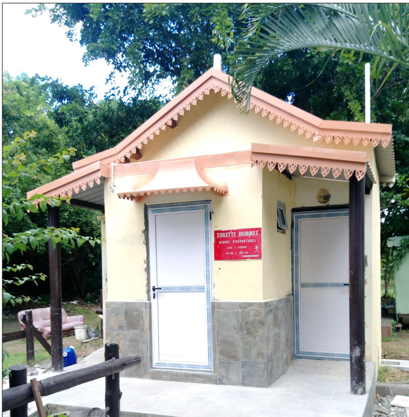
Painting of roof structure, replacement of openings & laying of slate tiles for toilet block at Sable Noir public beach (work in progress)
