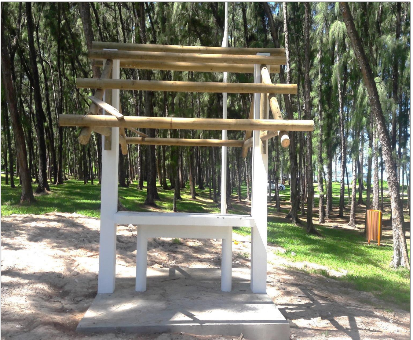
Construction of mini-kiosks at Pomponette public beach (works in progress)
