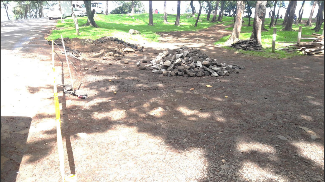
Upgrading of access at Rivière des Galets public beach (works in progress)
