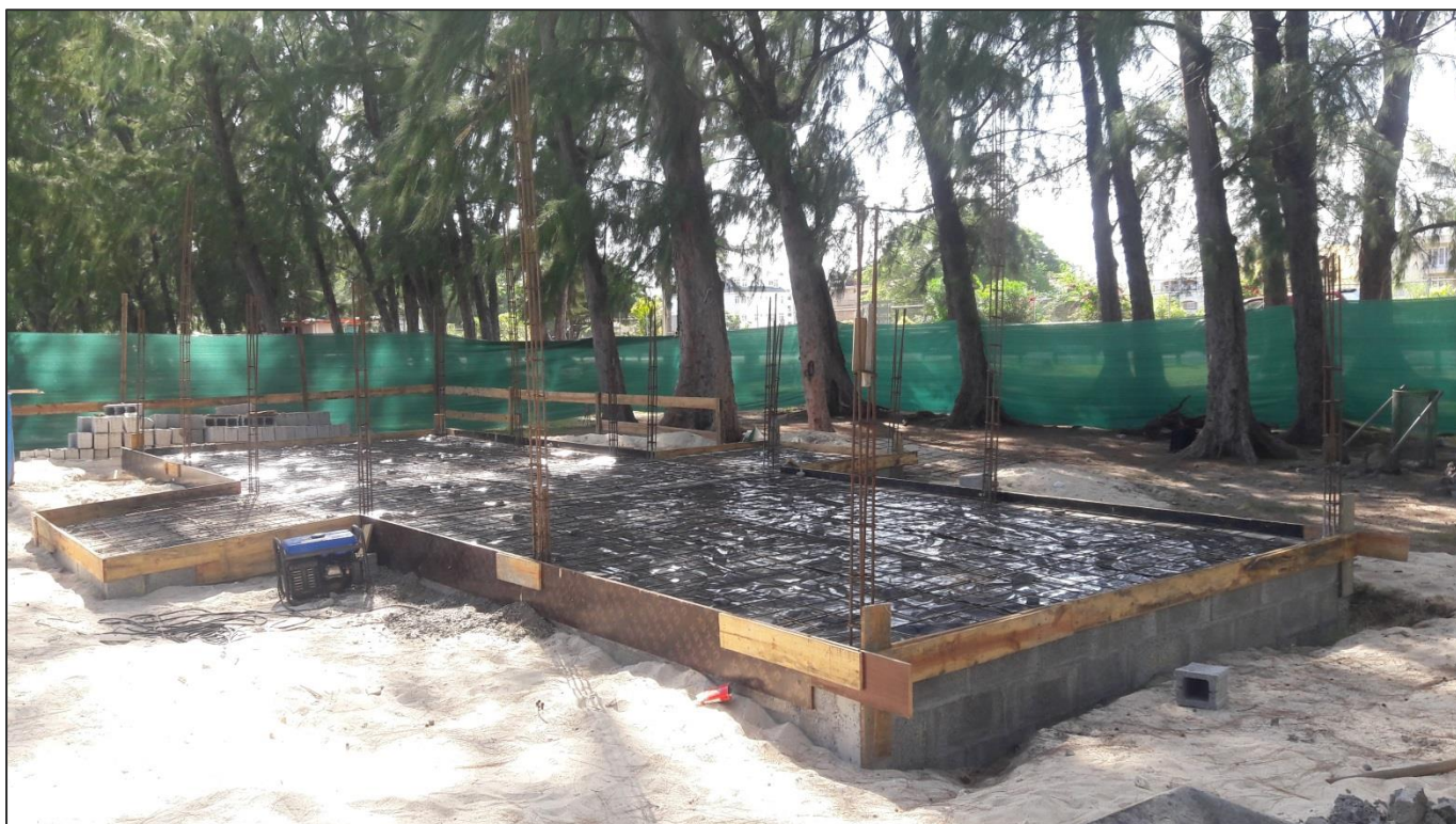
Sub structure works in progress for construction of new toilet block at Flic en Flac public beach (near Ex-Mer de Chine)
