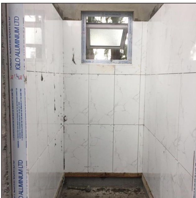
Laying of wall tiles Work in progress
