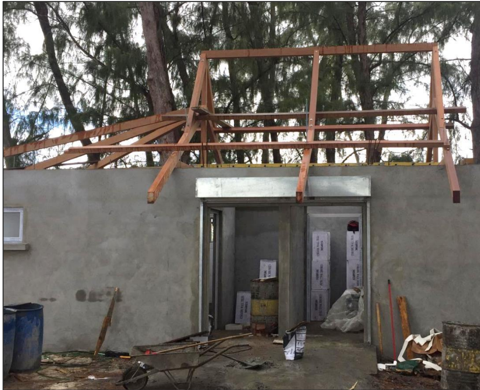
Wooden roof truss – construction in progress Fixing of anodised roller shutters
