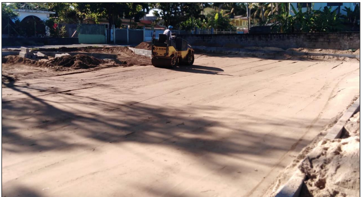
Levelling and compacting of parking area at Riambel public beach Work in progress
