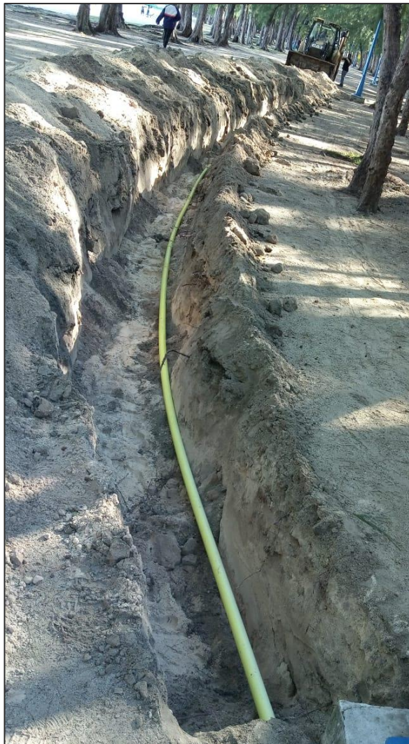
Laying of electric cables for relocation of CEB meter at Mont Choisy public beach
