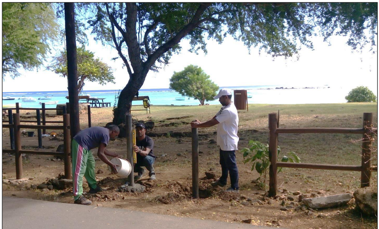
Replacement of damaged parapet wall at P. G. Anna public beach Work in progress
