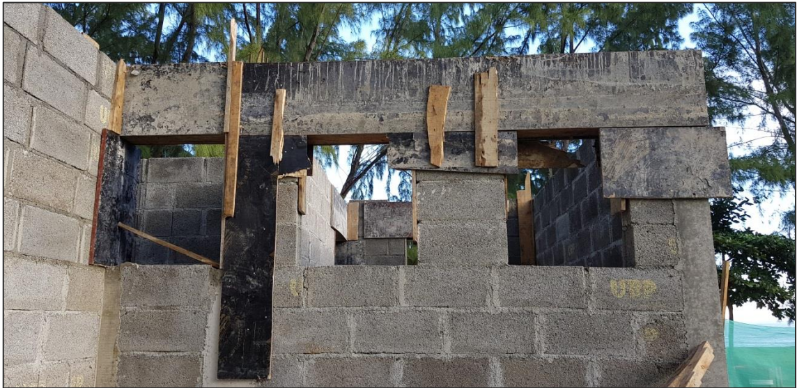
Construction of new toilet block at Riambel public beach Laying of blocks - work in progress
