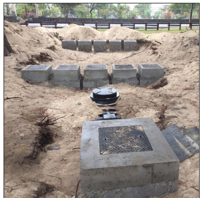
Fixing of manhole cover Work completed
