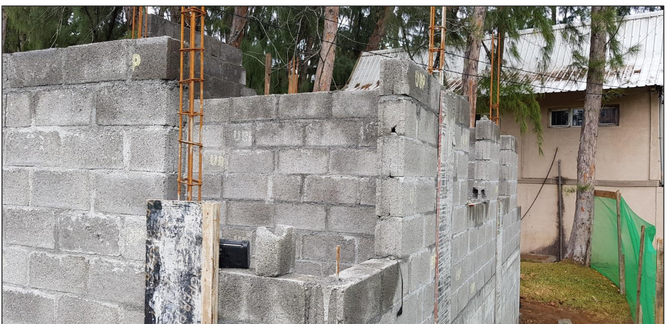
Construction of new sub office at Saint Felix public beach (laying of blocks and casting of columns ongoing)
