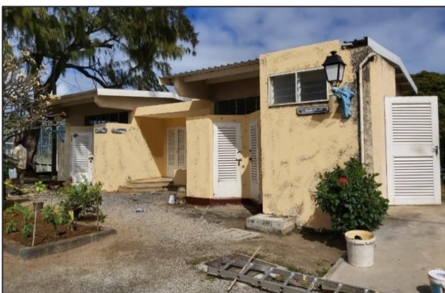
Painting of toilet block - Before
