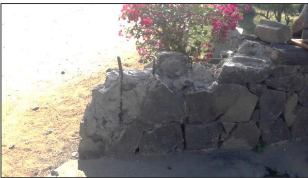
Reinstatement of masonry wall - Before
