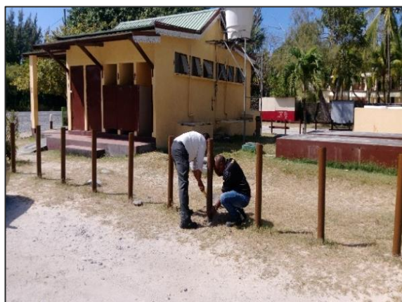
Painting of toilet block and bollards Before
