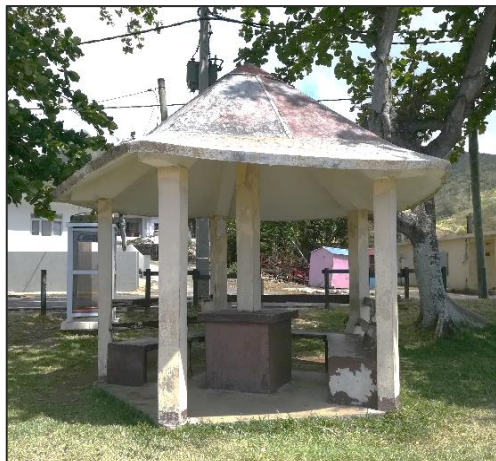
Painting of kiosk and refurbishment of bench - Before
