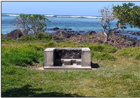
Reinstatement and painting of fireplace - Before
