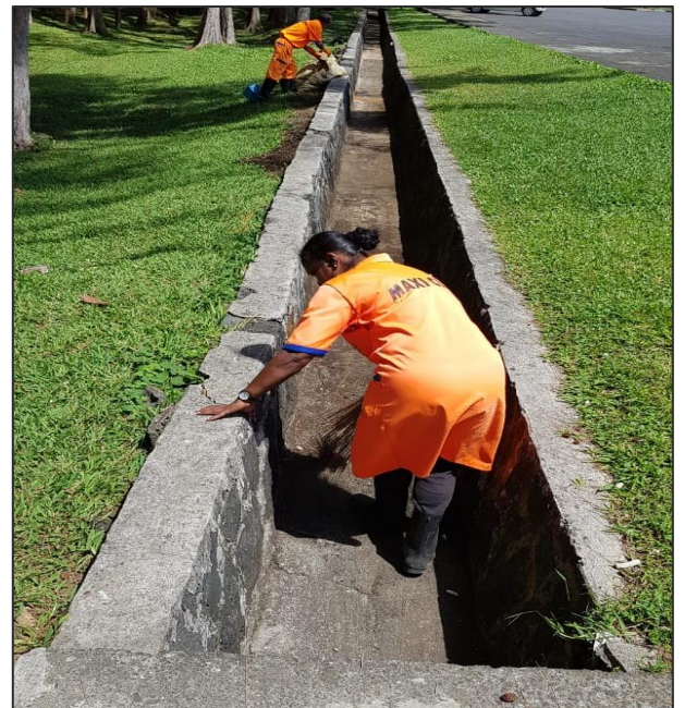
Cleaning of storm water drain
