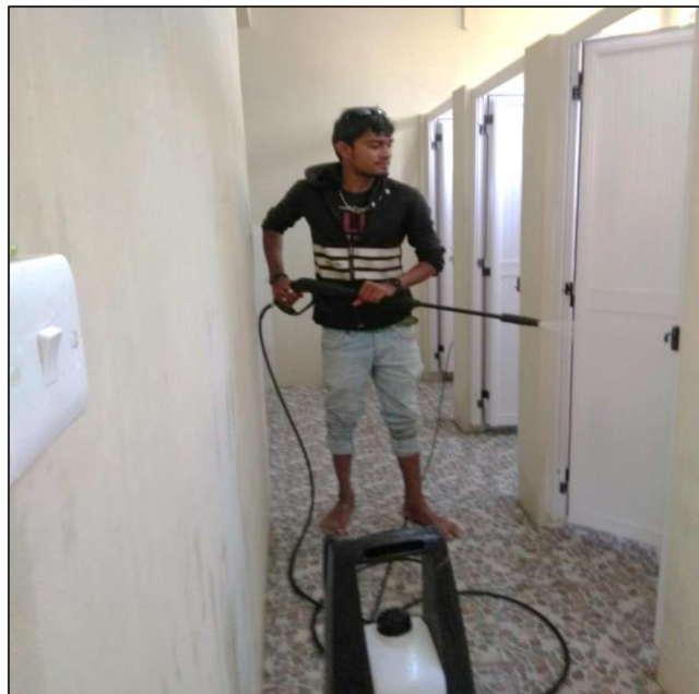
Toilet Block at Belle Mare public beach
