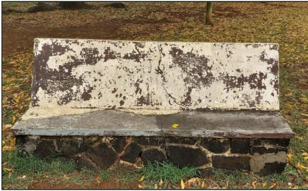
Painting of concrete benches Before
