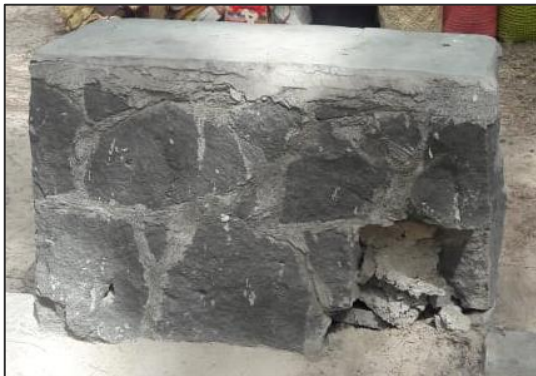
Reinstatement of stone masonry wall Before
