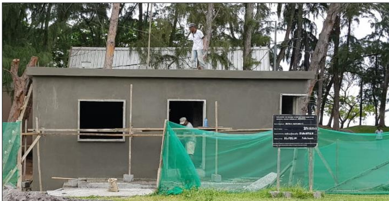
Plastering of external walls (Work completed)
