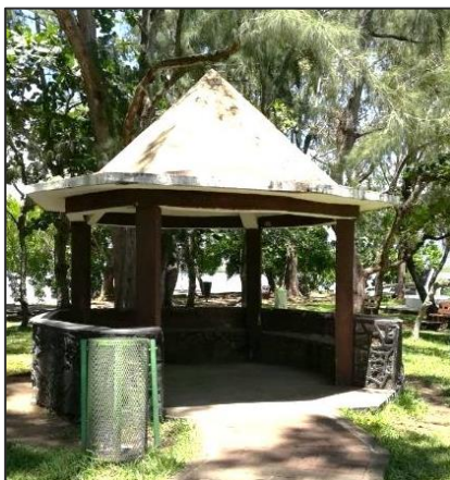
Painting of kiosk and bin - Before
