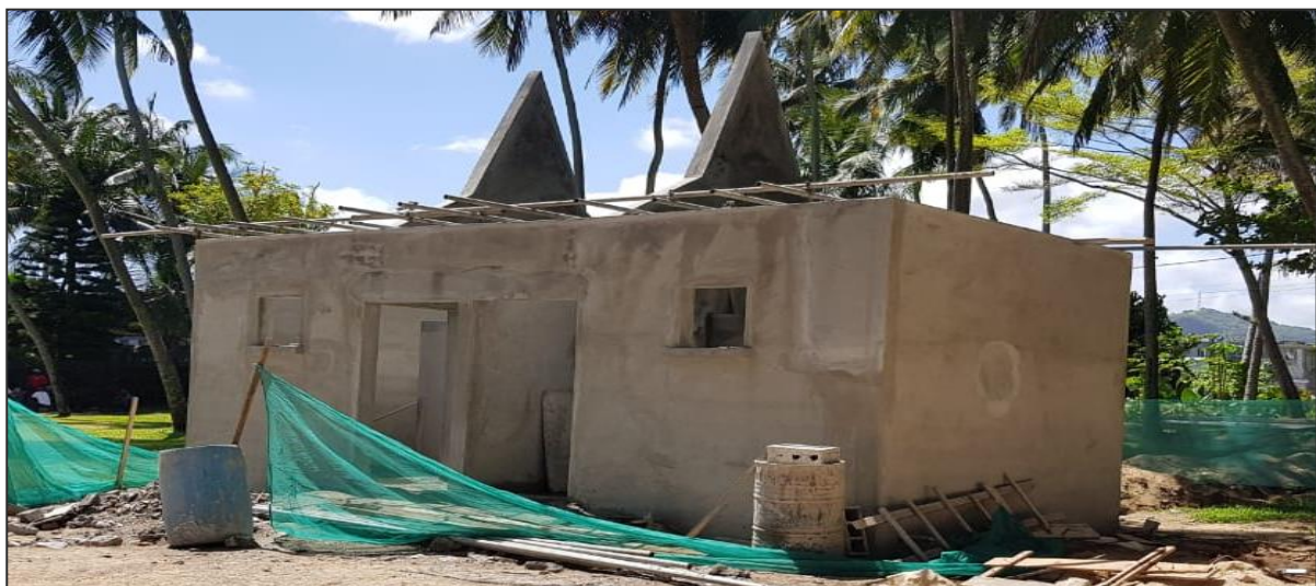
Construction of a new toilet block at Riambel public beach (Work in progress)
