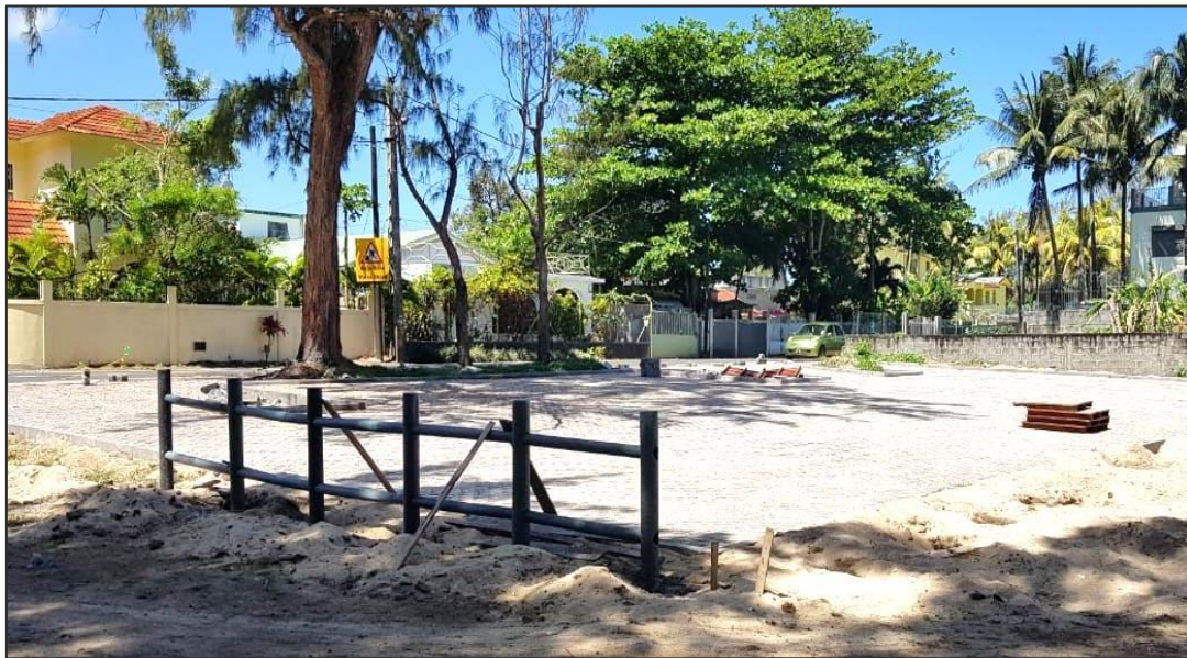
Laying of ecoblocks and backfilling with crushed corals (Work completed)
