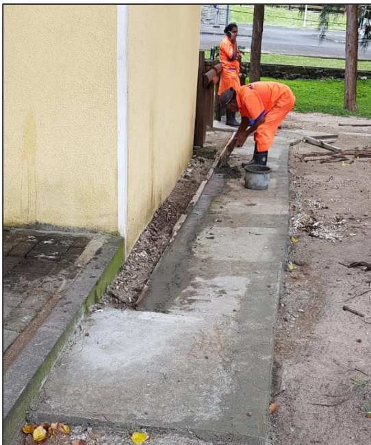
Maintenance of concrete footpath
