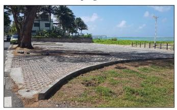
Laying of ecoblocks and backfilling with crushed corals (work completed)
