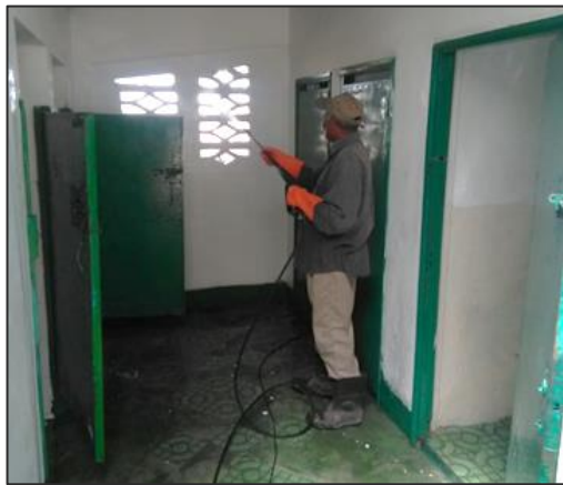
Toilet block at Poste Lafayette public beach
