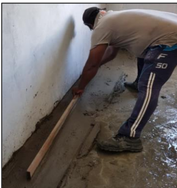
Placing of mortar for floor tiles
