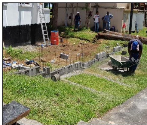
Construction of reinforced boundary wall
