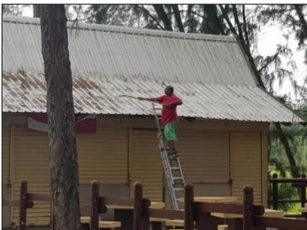
Cleaning of roof of tuckshops
