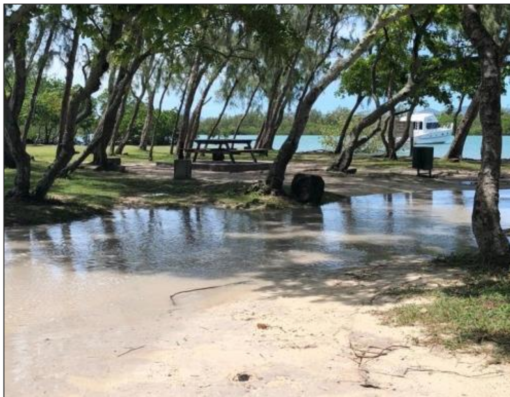
Accumulated water ingress at Bras d'Eau public beach
