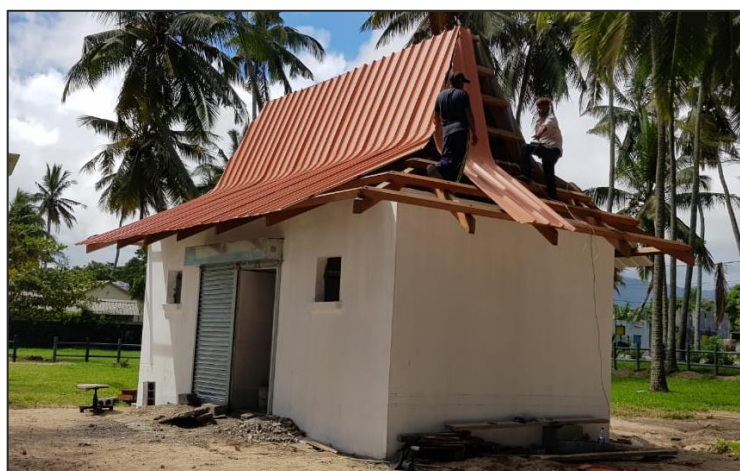
Construction of new toilet block at Riambel public beach (work in progress)
