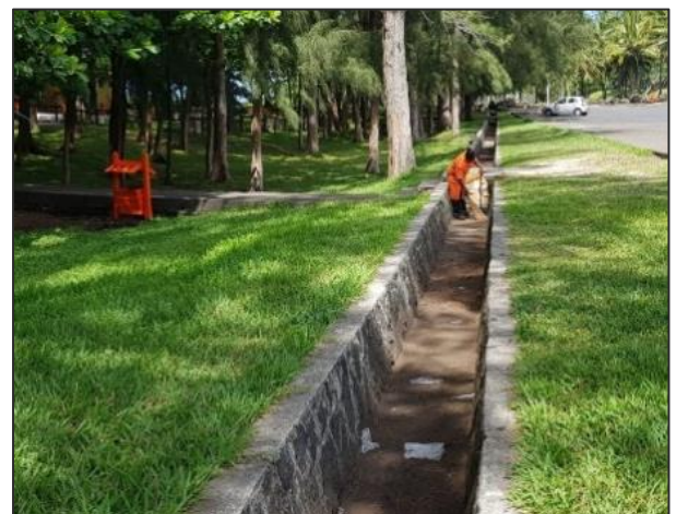
Cleaning of storm water drains
