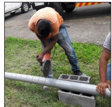
Preparation of sewerage perforated pipe
