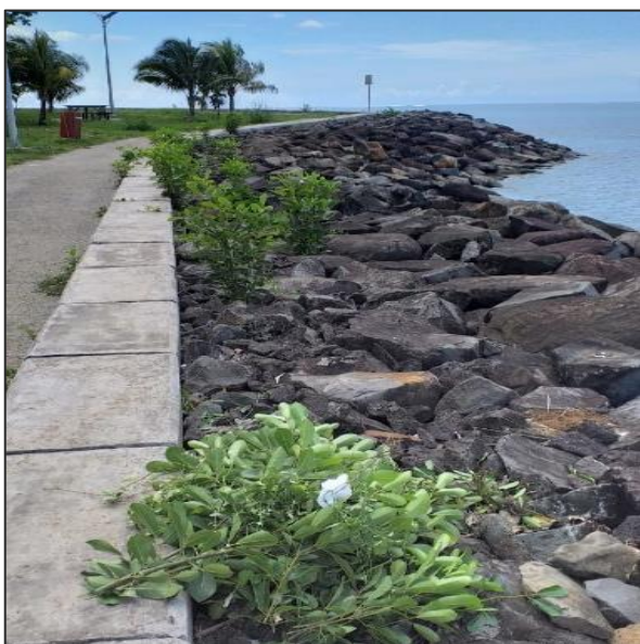
Maintenance of rock revetment - Before
