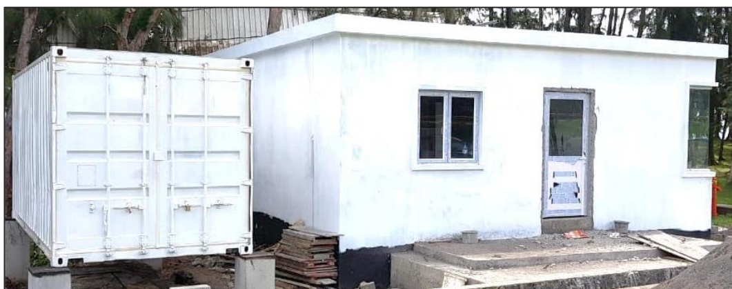
Rendering and installation of openings – work completed
