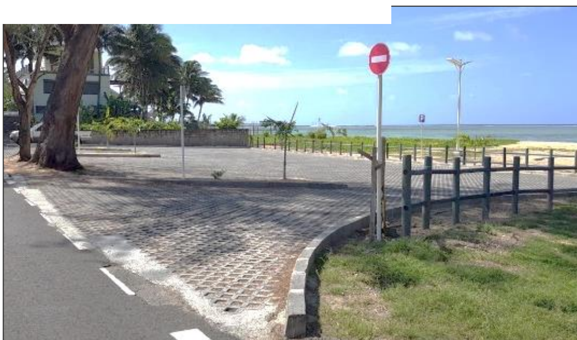
Construction of parking area – work completed
