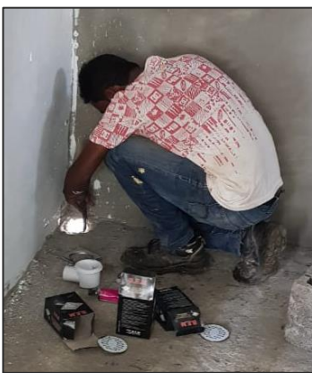
Installation of floor traps
