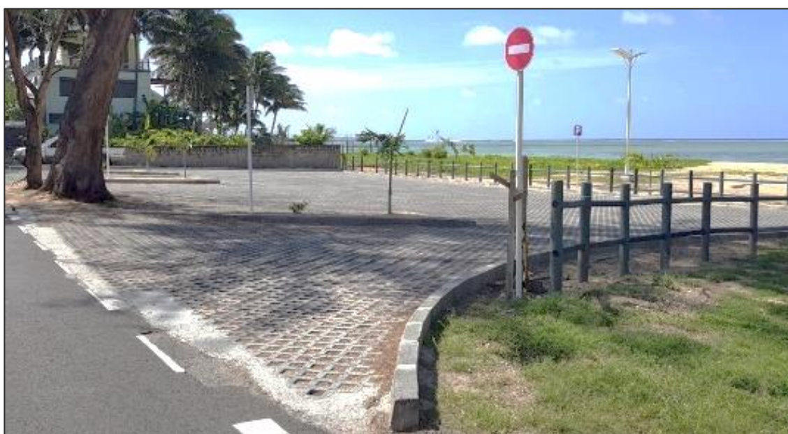
Construction of parking area – work completed
