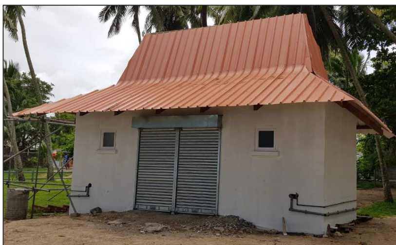
Construction of new toilet block at Riambel public beach (work in progress)
