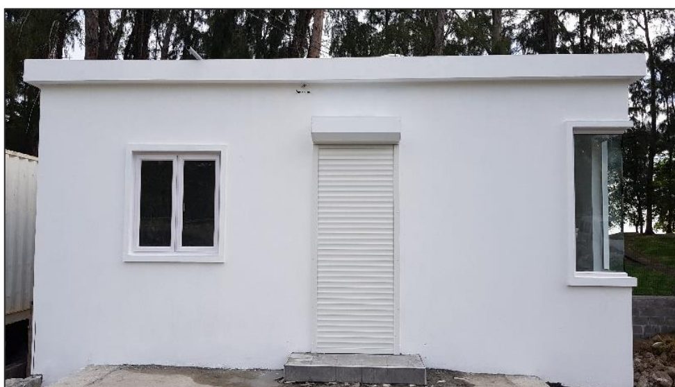
Installation of openings and fixing of roller shutter – work completed
