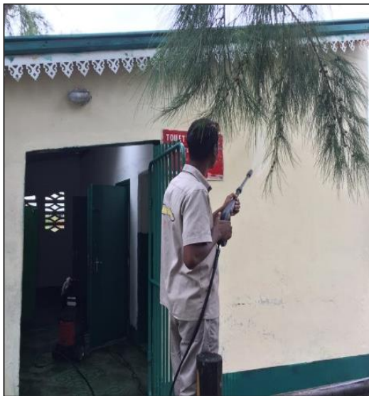
Toilet block at Belle Mare public beach
