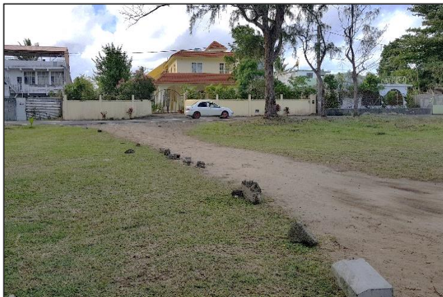
Construction of parking area - Before
