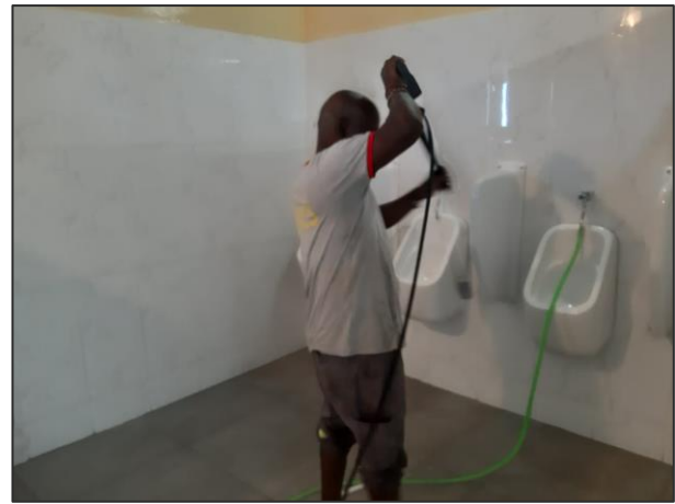
Toilet block at Flic en Flac public beach
