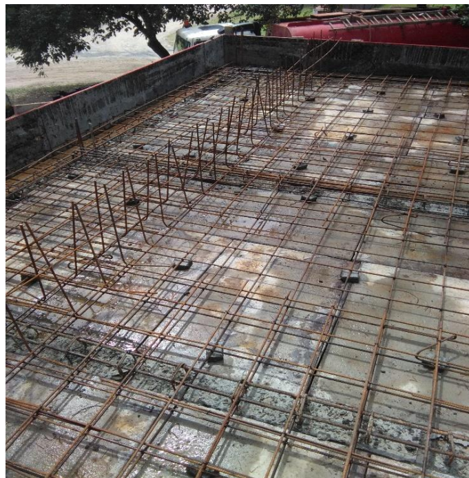
Preparation for casting of slabs
