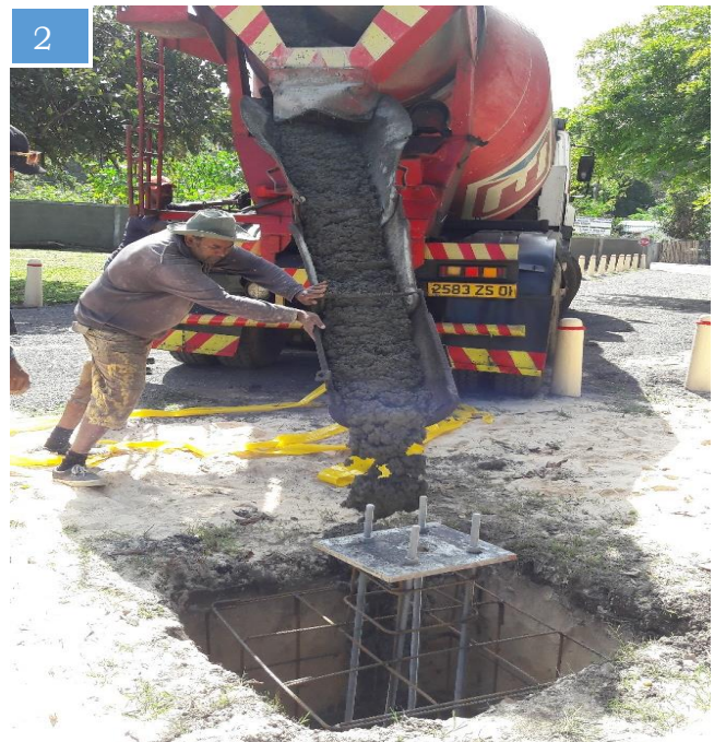
Casting of concrete column base
