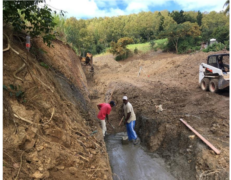
Casting of retaining wall base
