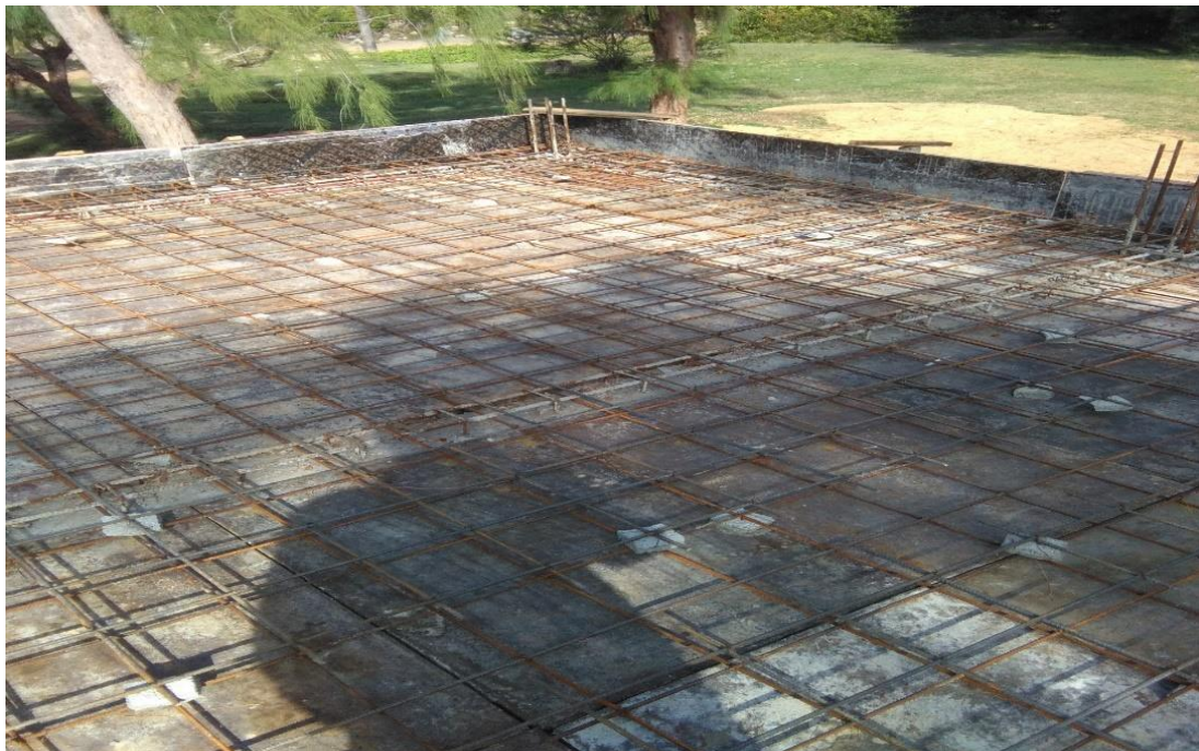
Preparation for casting of slabs
